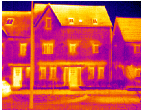
Stamford Brook, thermographic image
