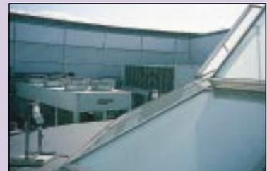
Condensors installed to serve the computer room chillers are located very close to the inlets serving the office chiller.
