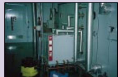
One of the rogue humidifiers which often runs in summer to replenish the moisture that is removed at the cooling coil.
