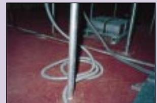
Lighting ballasts in the floor plenum are believed to be responsible for a 1°C hike in supply air temperature.
