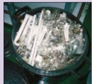
Evidence of the high rate (in reality up to 40 every month) at which the metal halide lamps need to be replaced. Each lamp costs £25.
