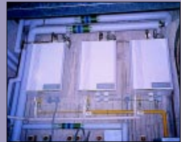
The total normalised gas consumption for the Elizabeth Fry Building in 1997 was measured at 37 kWh/m 2 /y, one fifth of the academic building low benchmark.
