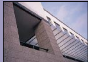
Some areas were initially underheated, like this first floor corner room above a walkway.
