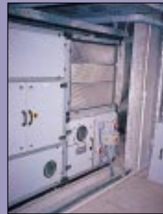
The heat recovery systems for two of EFry's air handling units use high-efficiency heat exchangers. These are claimed to recover 85% of the available heat, a figure verified by the monitoring.
