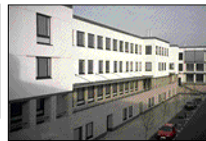
#14 FRY The Elizabeth Fry Building
