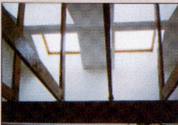
The inaccessible Velux windows have never been opened, causing overheating and...
