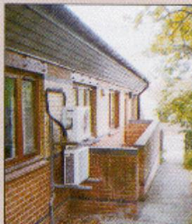
...the inevitable but excusable response: dx coolers bolted on to the outside of a green building. Despite provision for passive stack ventilation, the building users took the fit-and-forget route to solving their problems.
