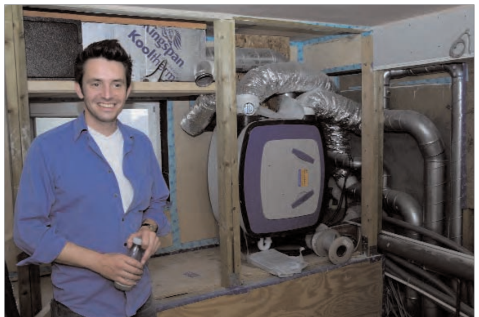
Above: Architect Robert Prewett with 89 Culford Road's Itho HRU Eco 4 mechanical ventilation with heat recovery unit. This is said to possess a reclaim efficiency of up to 91 per cent, predicted to give a cut of 4264 CO 2 kg per annum compared to the dwelling's original heat requirements.
