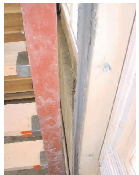
Above: An internal frame was constructed inside the front wall to support rebuilt floors and also to eliminate thermal bridges. The gap between the existing façade and the frame is filled with 140 mm of insulation.
