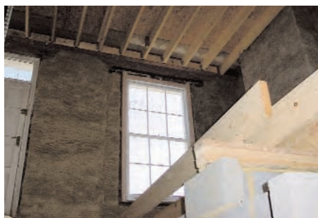
Above: The front wall rendered and awaiting insulation.
