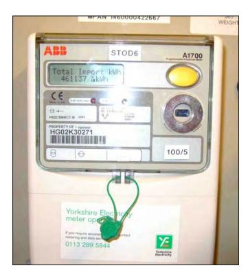
The rincipal sub-meter was not working, so the utility meter fault went five years undetected. The other two were wrongly calibrated, so impossible to do cross checks.
