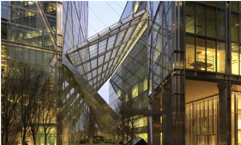
Figure 2 View of covered galleria between 201 Bishopsgate and the Broadgate Tower (201 Bishopsgate on right)
