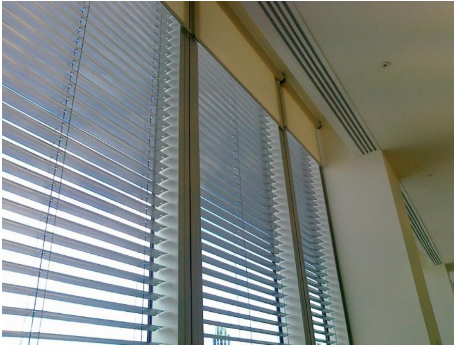
Figure 27 internal view of façade showing mullions and blinds
