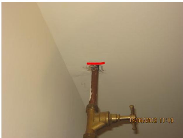
Cold water pipe from loft space penetration unsealed. Flat B in head of stairs cupboard.
