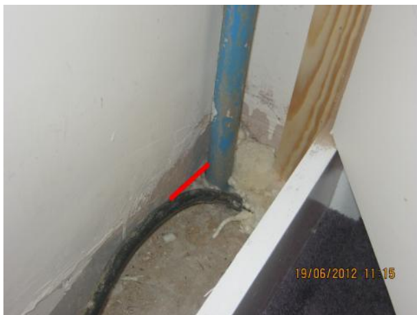
Foot of dry-lining unsealed at foot of stairs distribution cupboard and breaks in the dry lining at foot of stairs cupboard.
