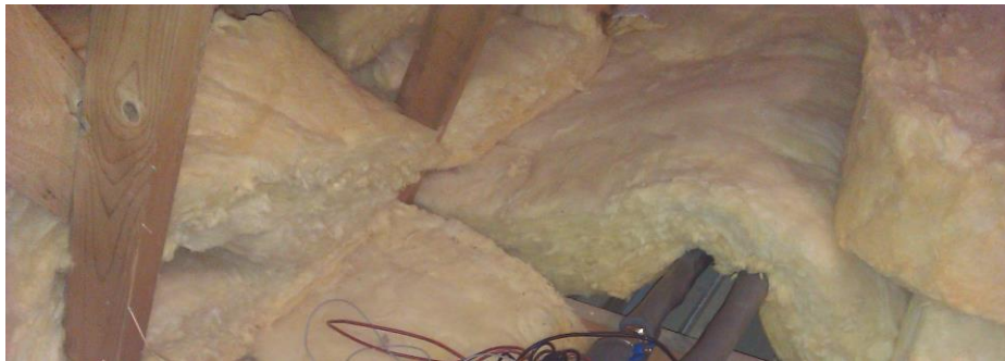
Figure 10: Loft insulation and heating & hot water pipes
