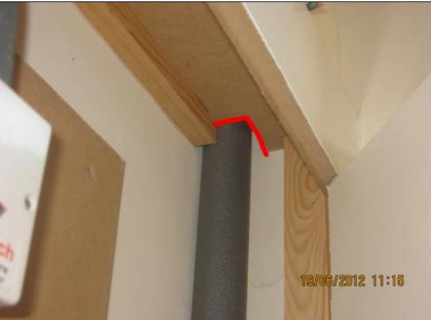
Unsealed boxing at foot of stairs distribution cupboard. Flat 15
