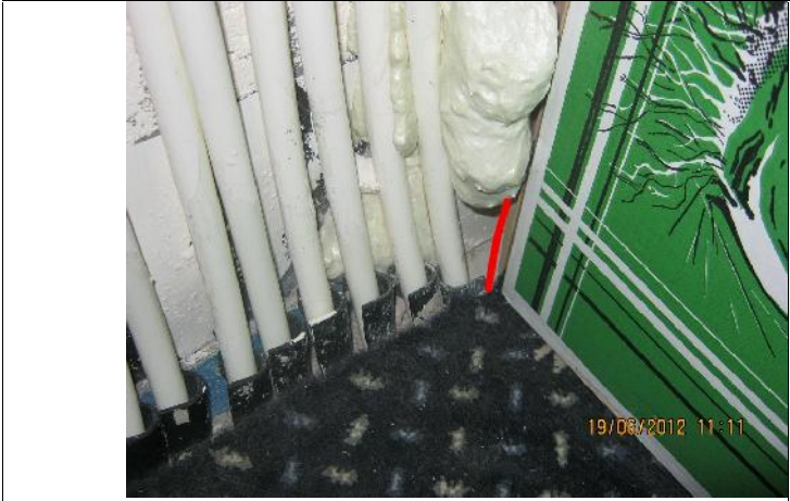
Boxing at under-floor heating manifold not sealed in flat 15 at head of stair cupboard.
