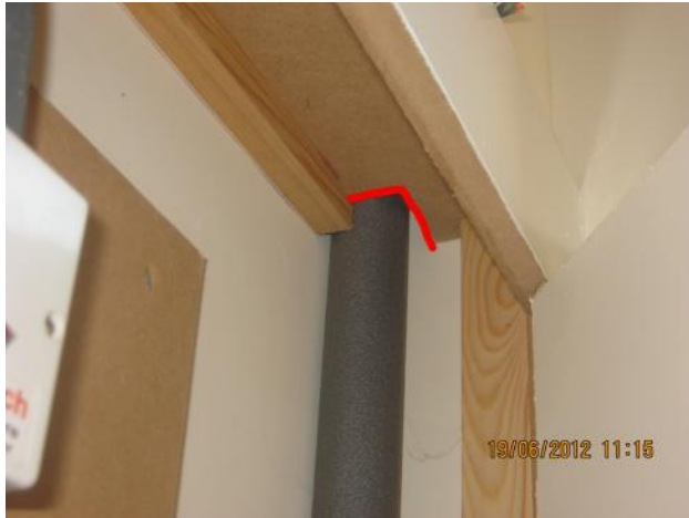
Unsealed boxing at foot of stairs distribution cupboard.
