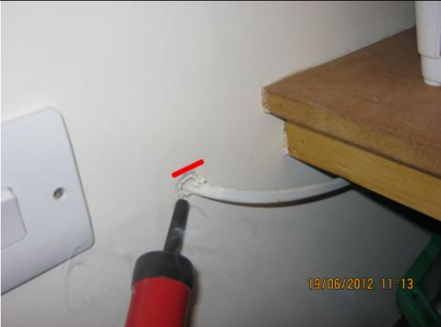
Cable penetrations into dry-lining unsealed. Flat 15 in head of stairs cupboard.
