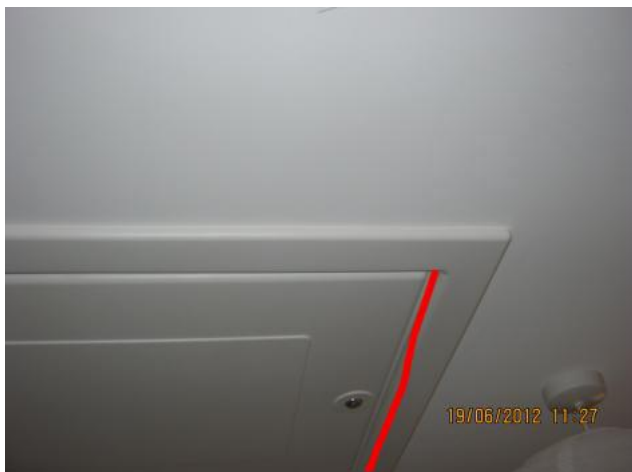
Loft hatches not sealing effectively allow flow of air into property from the cold roof space. Flat B
