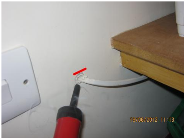
Cable penetrations into dry-lining unsealed. Flat B in head of stairs cupboard.
