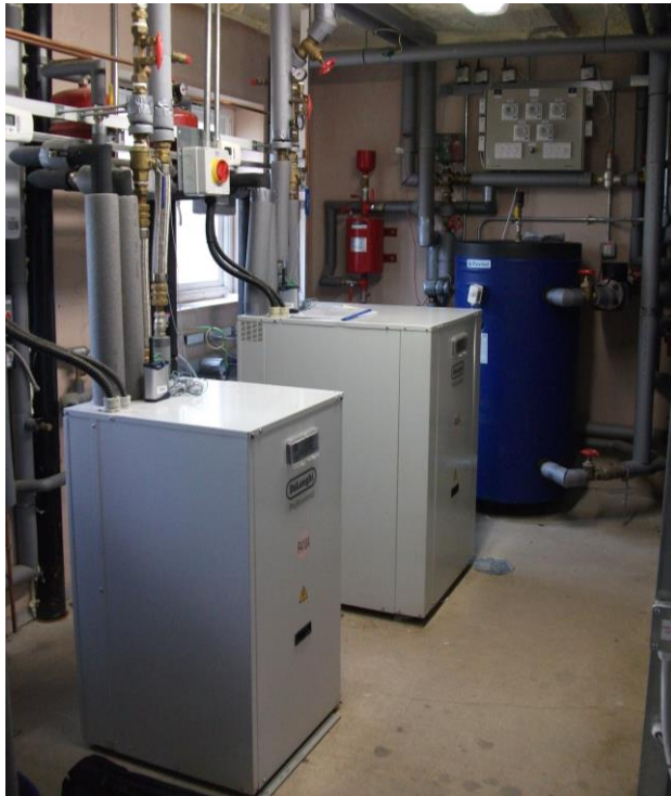
Figure 3: Photo of ground source heat pumps in the centralised plant room
