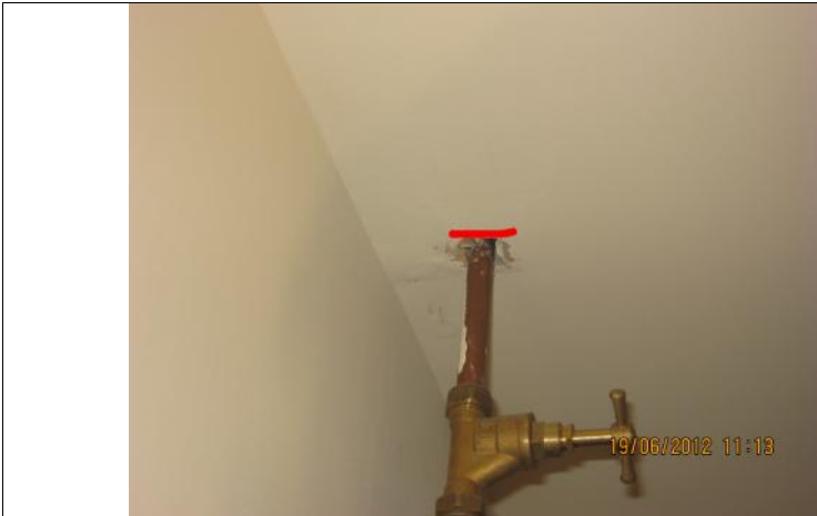
Cold water pipe from loft space penetration unsealed. Flat 15 in head of stairs cupboard.
