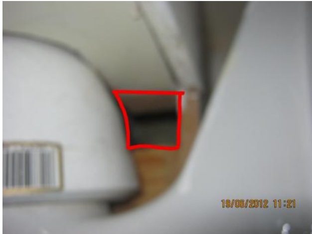
Toilet waste boxing unsealed again, in both flats allowing ingress.
