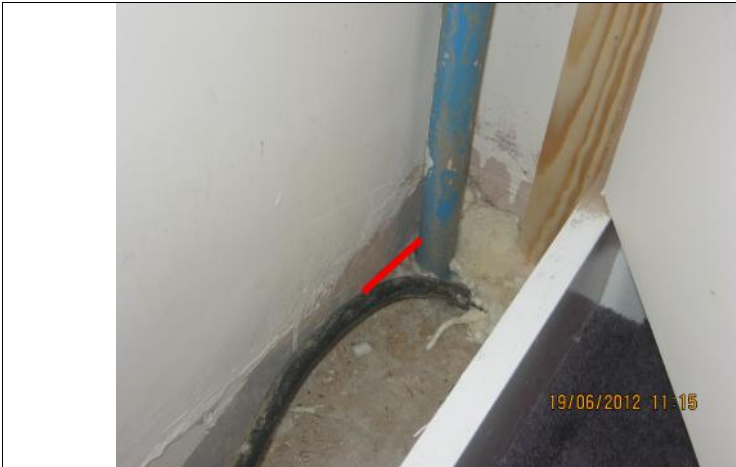
Foot of dry-lining unsealed at foot of stairs distribution cupboard. Flat 15
