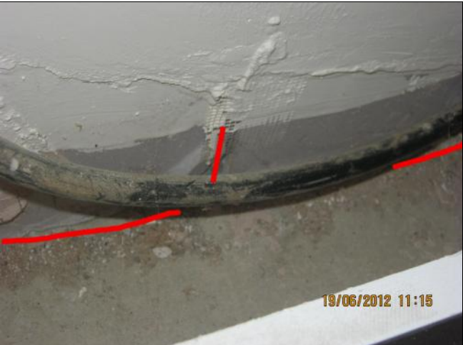
Breaks in the dry lining at foot of stairs cupboard. Flat 15
