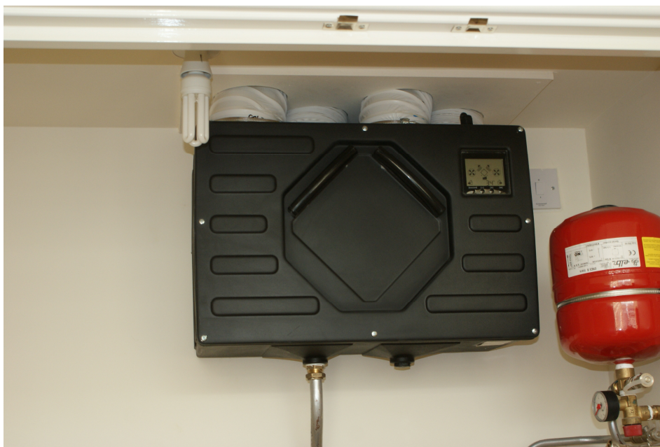
Photo 15 Greenwood HRV 1 unit with flexible ducting in airing cupboard
