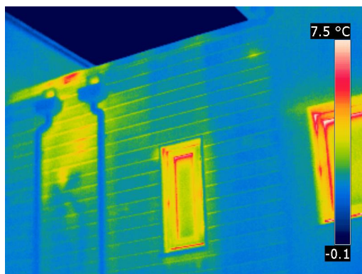
Photo 14 Outside rear elevation – party wall junction showing heat loss at parapet.
