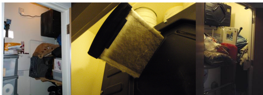
Photo 26 (left) narrow inaccessible cupboard with MVHR, photo 27 (centre) door frame clashes with filter, Photo 28 (right) MVHR cupboard as storage
