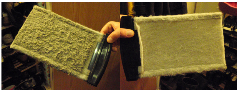
Photo 25 MVHR filter as found (left) and after cleaning (right)
