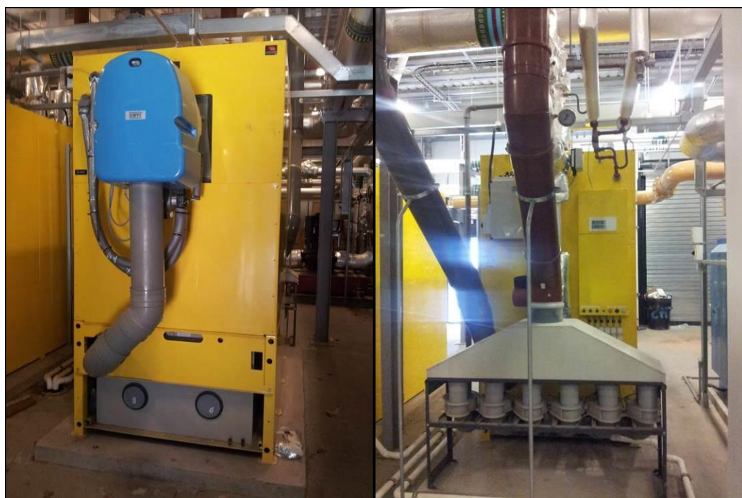
Figure 4 – Atlantic biofuel boilers
