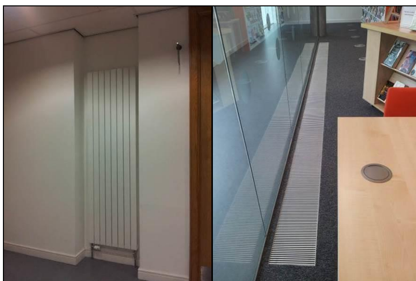
Figure 7 – Examples of heating provision; a radiator in the basement's corridor and trench heater in the library
