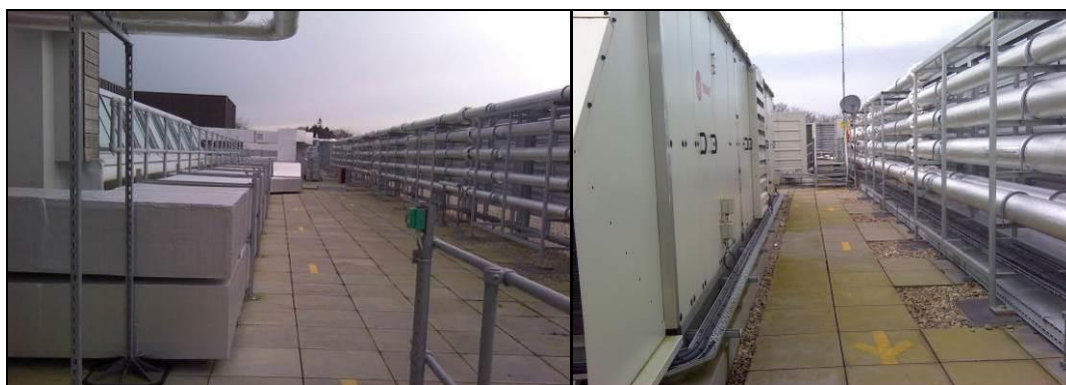
Figure 14 – Images of roof top plant; air ducts, an air handling unit and water pipes
