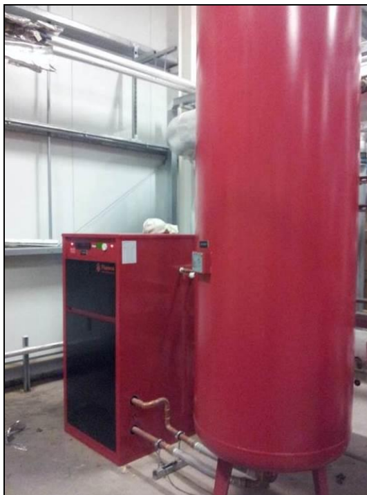
Figure 5 – Flamco Pressurisation unit
