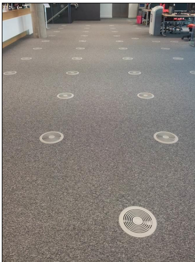
Figure 12 – Movable floor diffusers in the library
