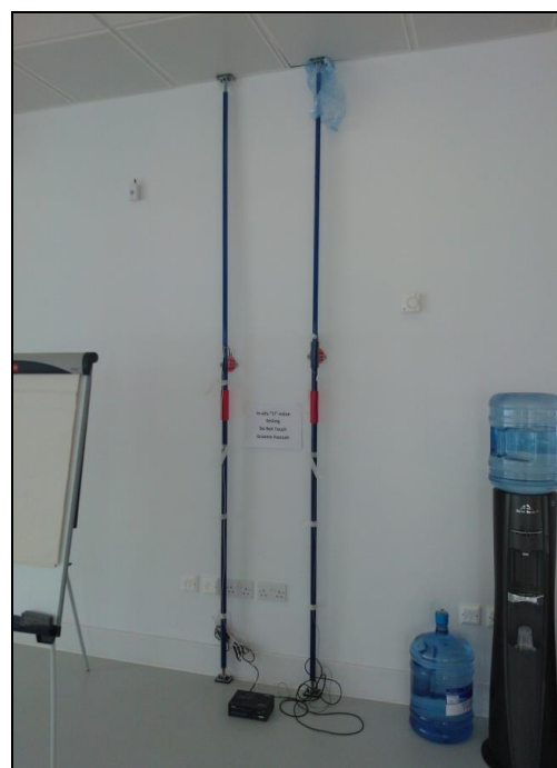
Figure 57: Heat Flow Meters
