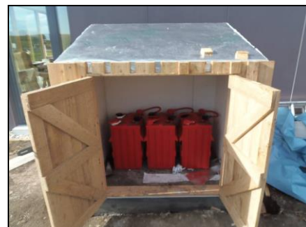
Figure 10: Battery Enclosure
