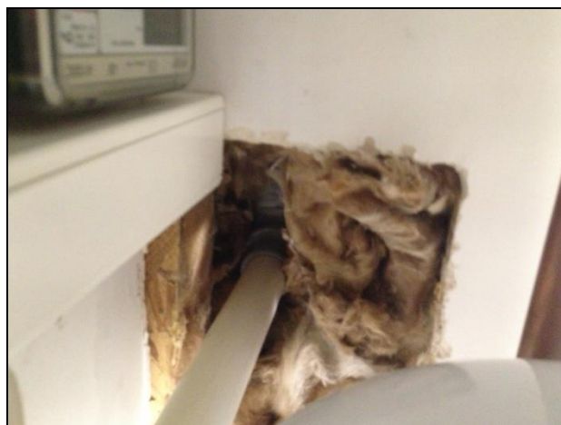
Figure 70: Break through Insulation (Wall)
