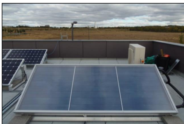
Figure 11: Solar Thermal Flat Plate Collector
