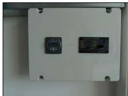
Figure 9: Battery Monitor
