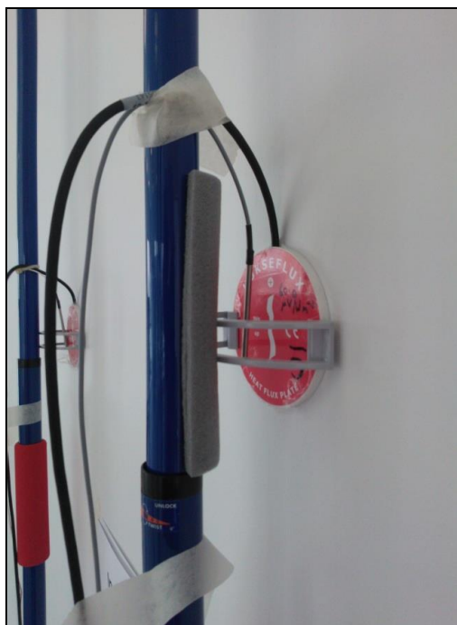
Figure 56: Heat Flow Meters
