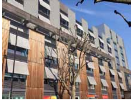
Above: External motorised blinds formed part of the integrated environmental design strategy.
