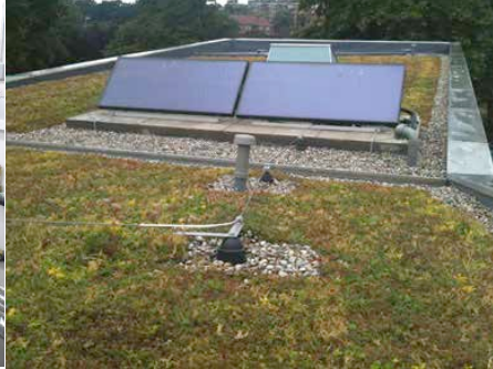
Fig.3.2.4 The roof mounted Solar Thermal Panels on New Building
