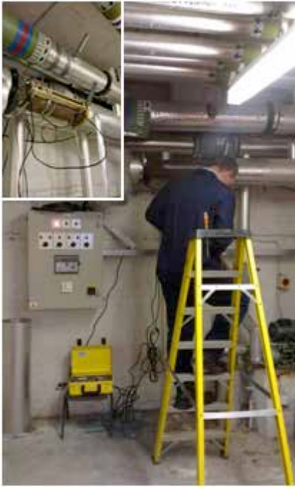
Fig. 6.3.2 – Installation of ultrasonic ‘clamp-on’ heat meters as part of two-year energy performance monitoring. Following temporary removal of a small section of pipework insulation, the meter is clamped to the outside of a straight section of bare pipe to measure flow rate, with temperature probes on flow and return pipes.
