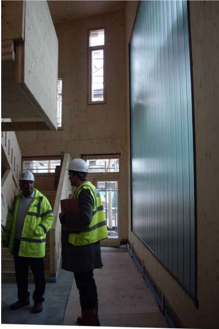
Fig.2.12.4- March 2010: Photo showing Reglit glazing and Rational window installed.
