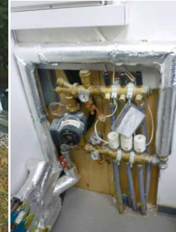
Fig.3.2.5 Heating manifolds in the New Building plant room
