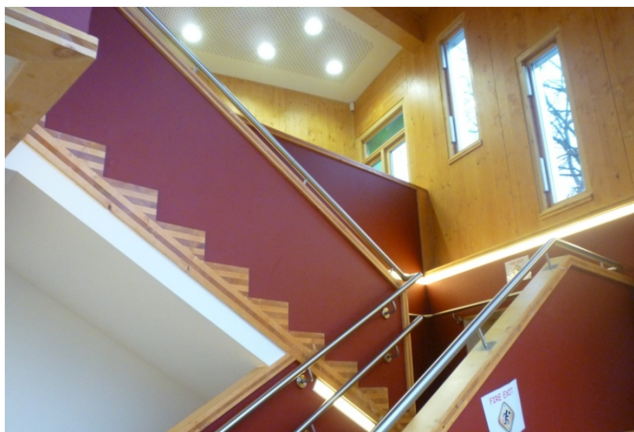
Fig 8.1.2 – Photo of feature lighting and ceiling lights turned on in the Children Centre's despite good daylight levels.
