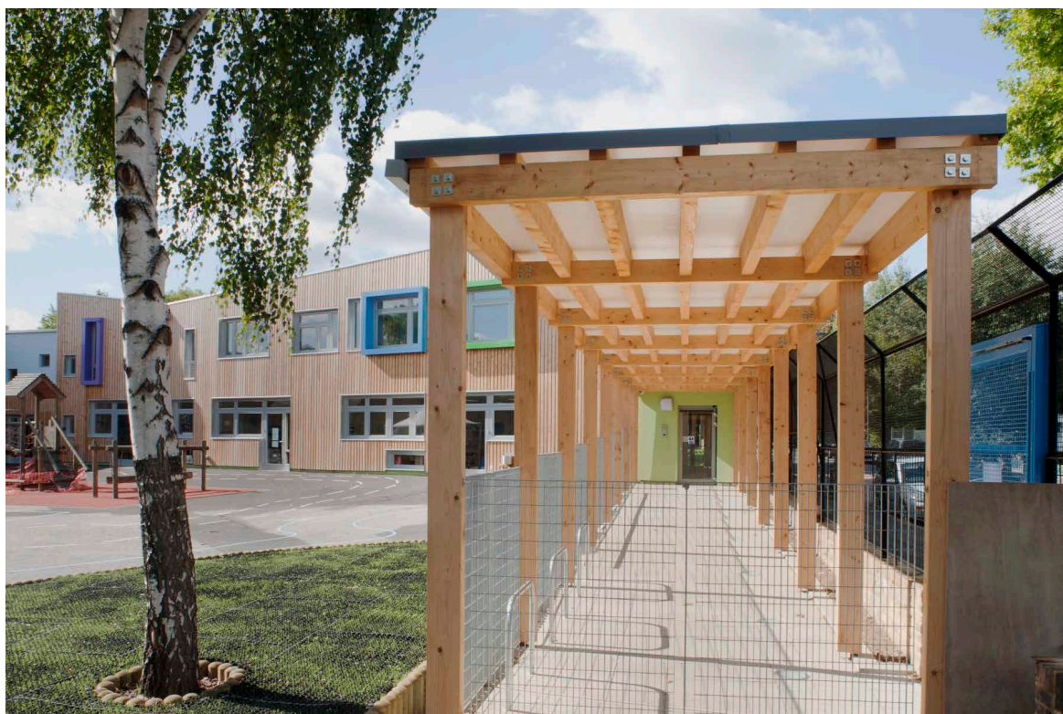
Fig.5.0.1 - The covered pergola to the Children's centre. This entrance provided an attractive and welcoming entrance to the building. Sheffield stands were fitted to allow visitors to secure buggies - however these were later considered insufficient and a separate store was retrofitted. See Fig.5.5.11.
