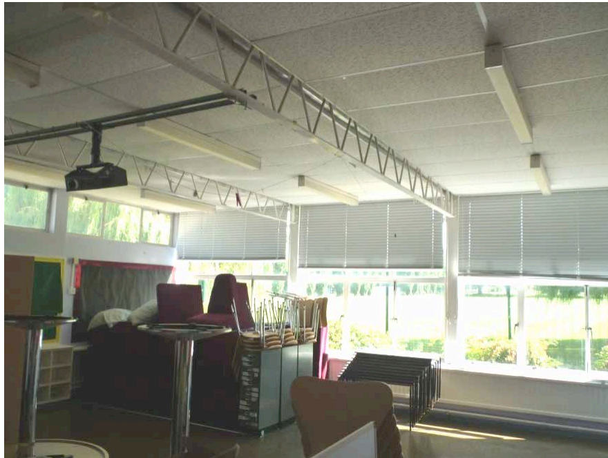
Fig 3.3.3 - Classroom windows in the Old Building
