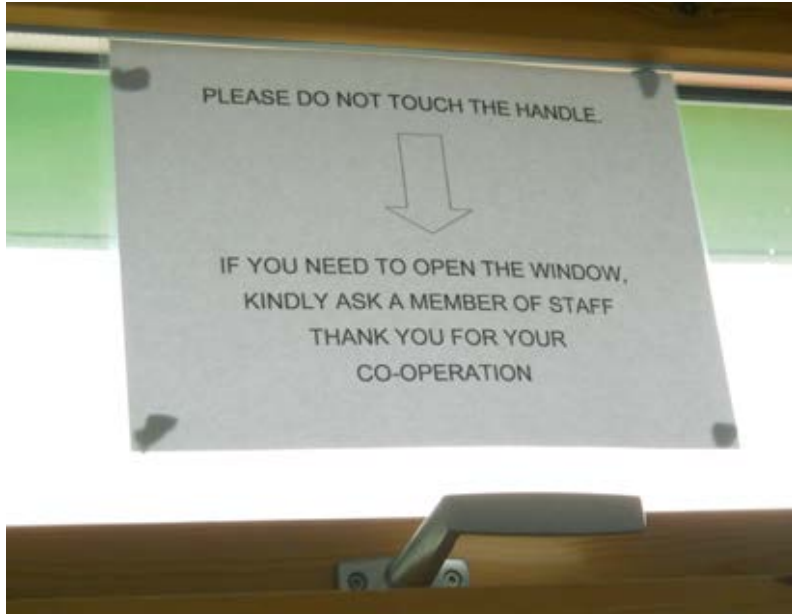
Fig 8.4.2 - Signage produced by the user to stop people incorrectly using the automatic window handle.
