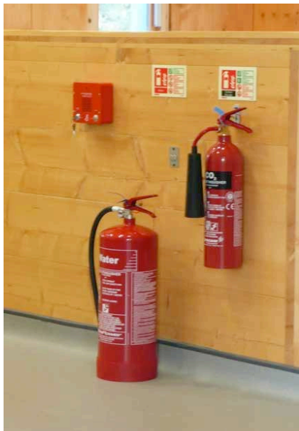
Keys left in the disabled refuge alarm
