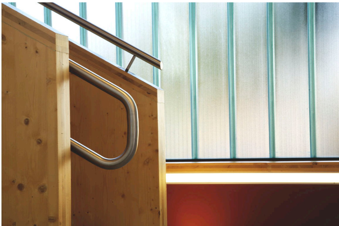
Fig.5.5.2- Photo of the Children Centre stair care 2012 – The palette of materials for the New Building included expressed cross laminated timber, natural lino cladding on walls, stainless steel and large windows for good natural light. The appearance of the building was highly prized by users.
