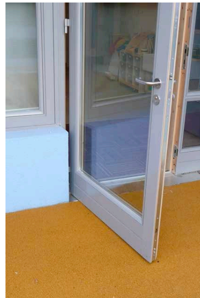
Fig 4.4.5 - Photo showing external doors prior to a friction stay being fitted.
