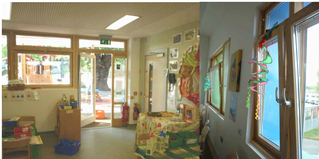
Fig 3.3.1– Doors and windows in the New Building ground floor classroom (left-hand image). New Building First floor windows showing restricted opening (right-hand image)
