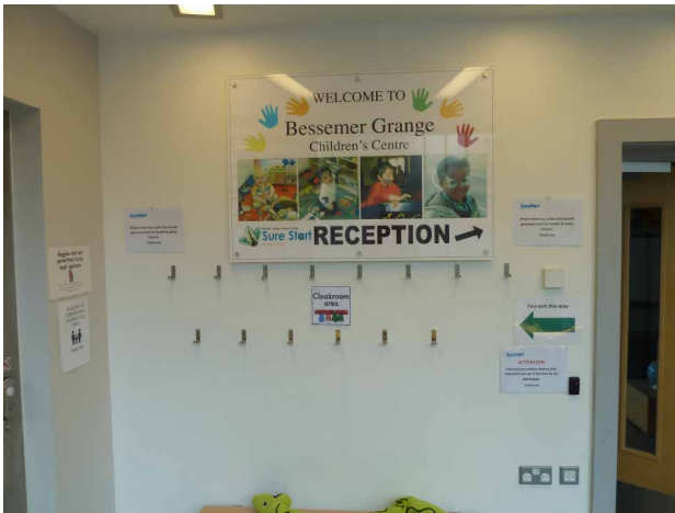
Fig.5.5.6 - Photo of the wall in the ground floor lobby of the Children's Centre. The design of signage was taken on by the client and not included in the main contract. This has led to a lot of unco-ordinated signs being fitted, which adds visual clutter to the spaces.
