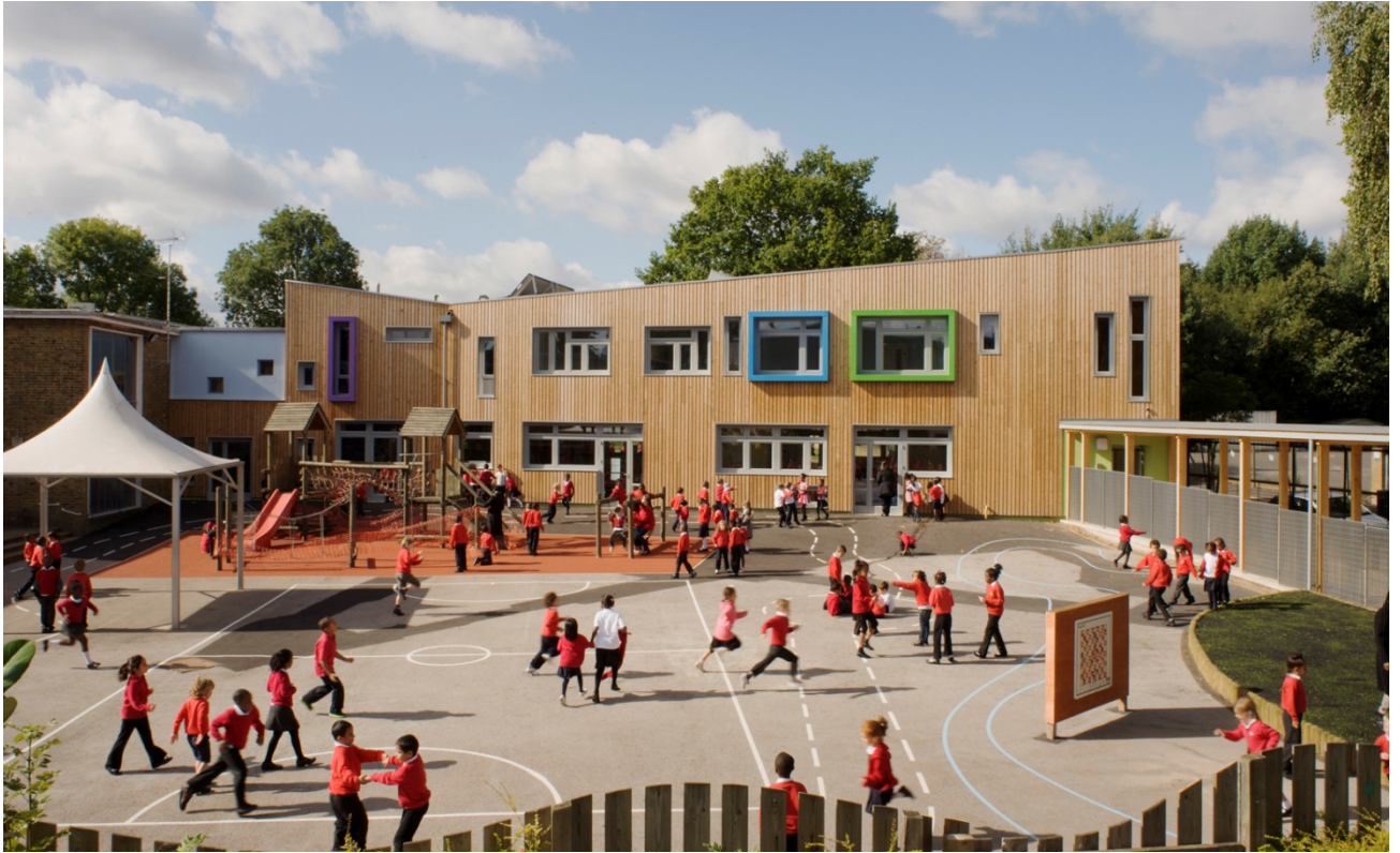
Fig.2.12.6- Photo of the completed New Building
