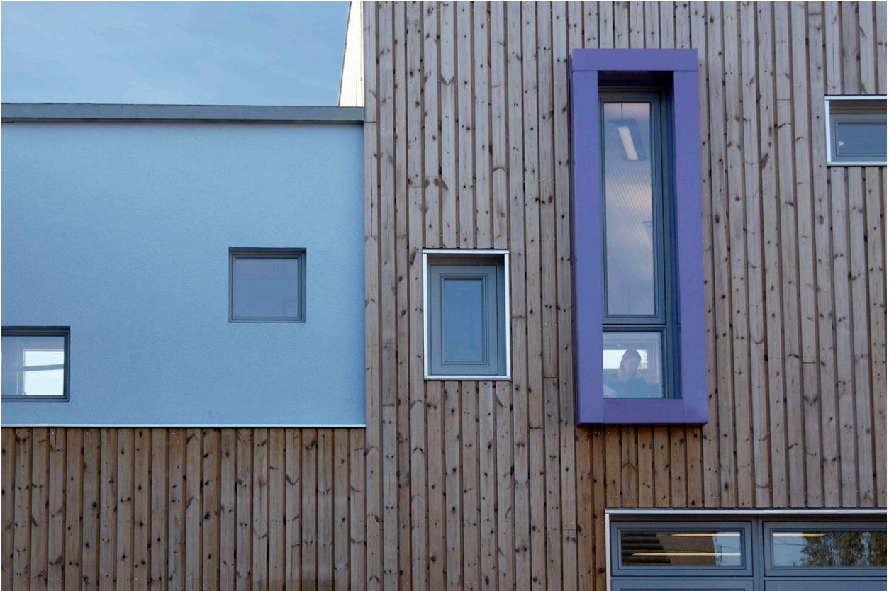
Fig 2.7.3 – A photo showing the expressed timber materiality of the project.
