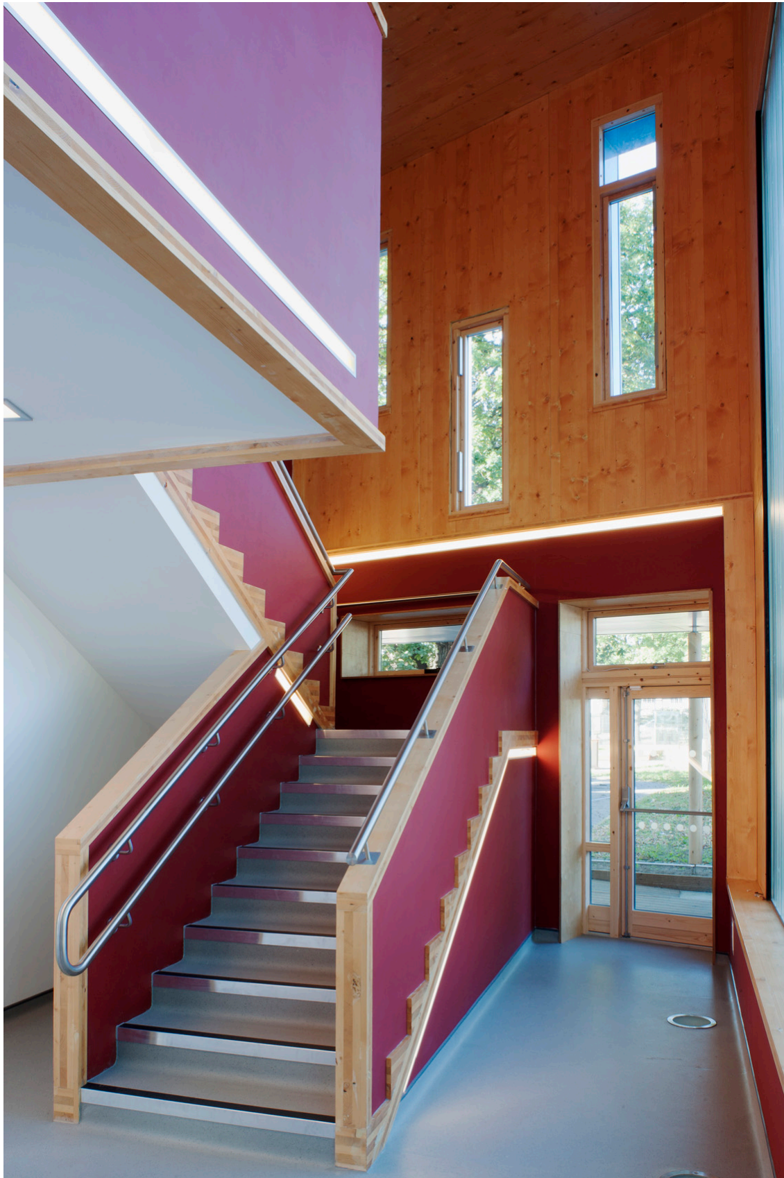
Fig.5.5.3- Photo of the New Building's feature staircase – 2012. This dynamic entrance which expresses the materiality of the construction helped create the New Building's positive image. However the new headteacher criticised it saying some features such as recessed lighting were expensive to maintain and were not sufficiently robust.
