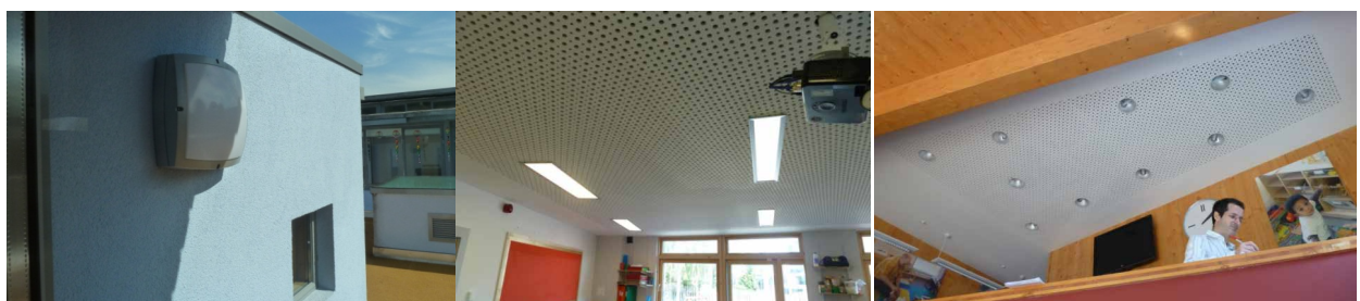
Fig 3.5.3 – Lighting in the New Building - left: low energy external lighting; Centre: ground floor classroom with acoustic ceiling and recessed T8 luminaires; right: high concentration of lighting fixtures in the first floor lobby/reception area
