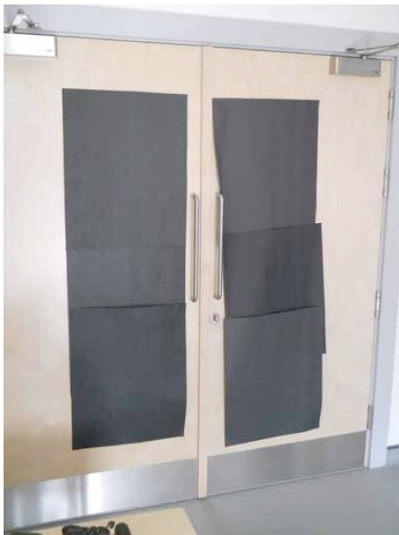
Fig 4.4.4 - Photo showing window covered up between the Crèche and training room.
