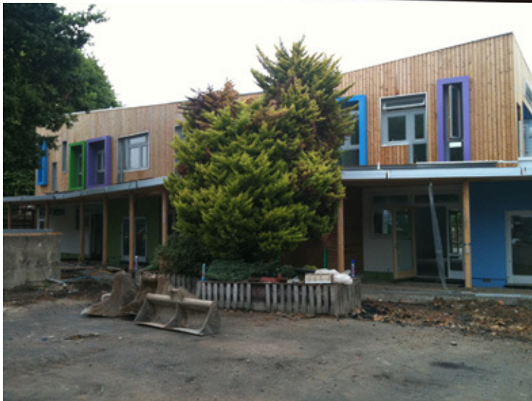
Fig.2.12.5- July 2010: Photo showing cladding completed. Landscape works progressing.
