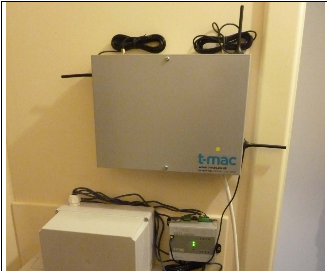
Fig.8.2 The t-mac 'gateway' unit. This collates the data from environmental monitors and sub-metered circuits and transmits wirelessly to t-mac technologies.
