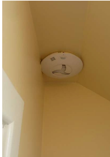
Figure 9.5: Inaccessible (for testing) WC extract fan
