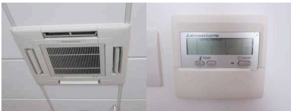
Figure 3-11 Comfort cooling indoor unit; comfort cooling controller
