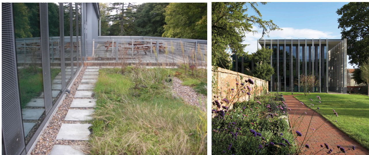
Figure 5: (Left) The green roof and external seating area
