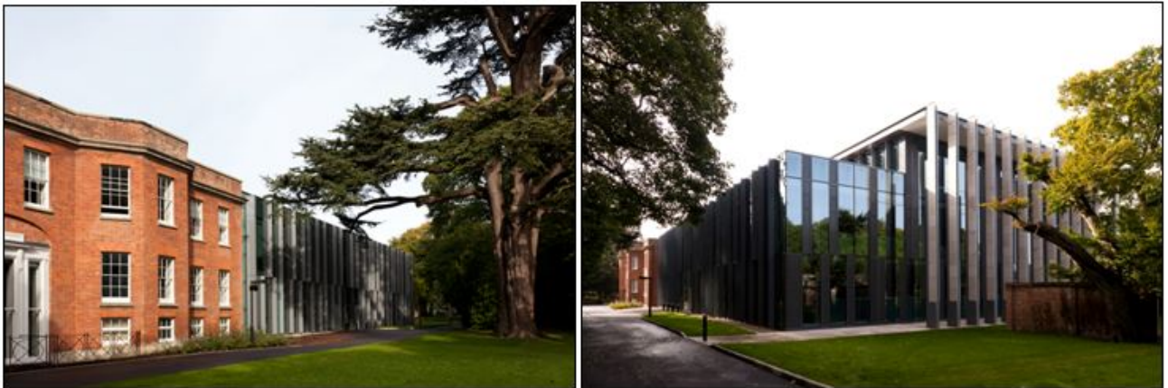
Figure 1: (Left) Photograph of the existing listed building and the new extension
