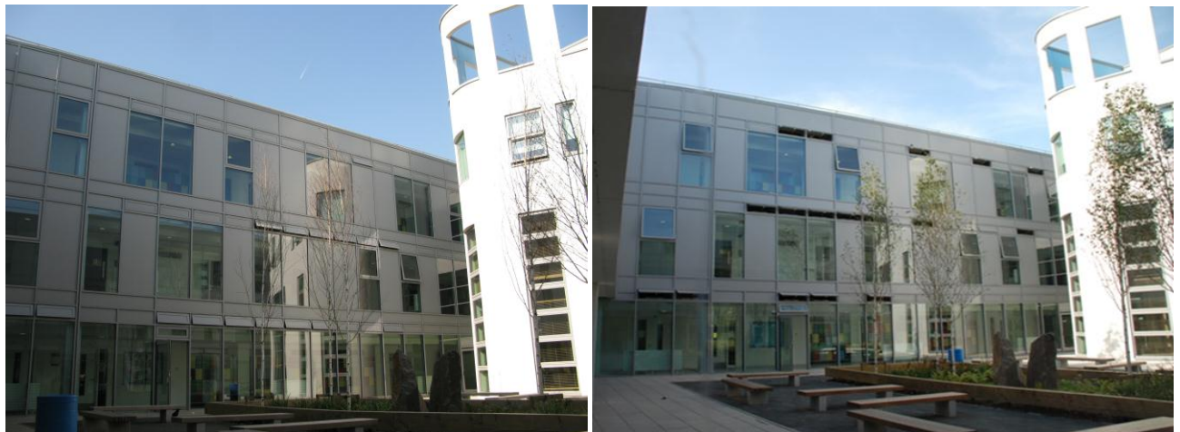
Figure 7.9: Winter and summer snapshot of West Wing and Classroom Pod showing 30% and 100% open plenum flaps respectively.
