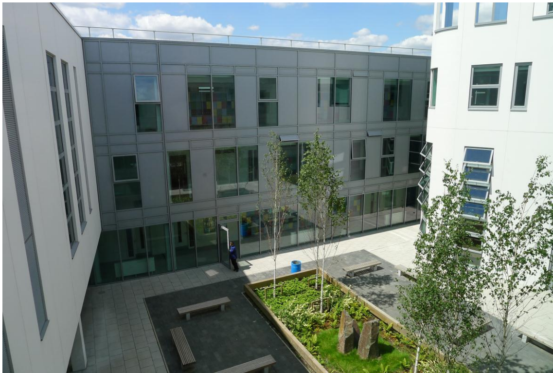
Figure 2.3: Loxford School Landscaped Courtyard and motorised vents embedded into the facades
