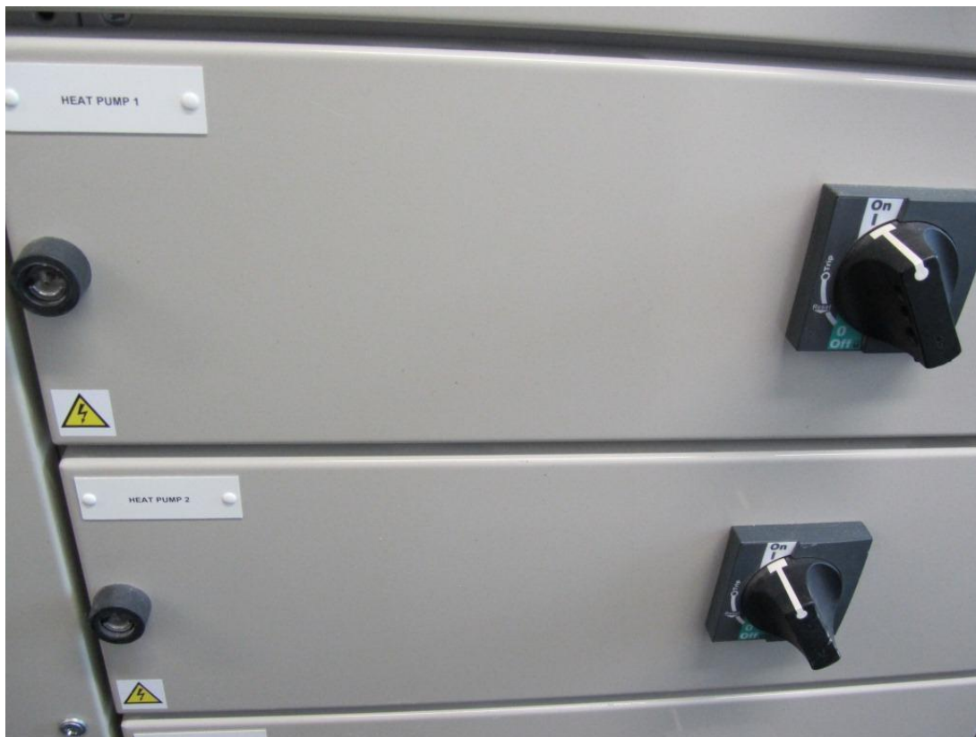
Figure 7.12: Heat pump electricity meters marked on LV panel but missing
