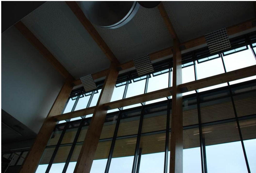
Figure 3.5: High-level vents in atrium spaces
