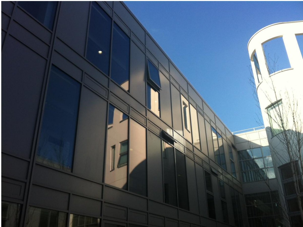
Figure 7.10: Plenum flaps stuck open
