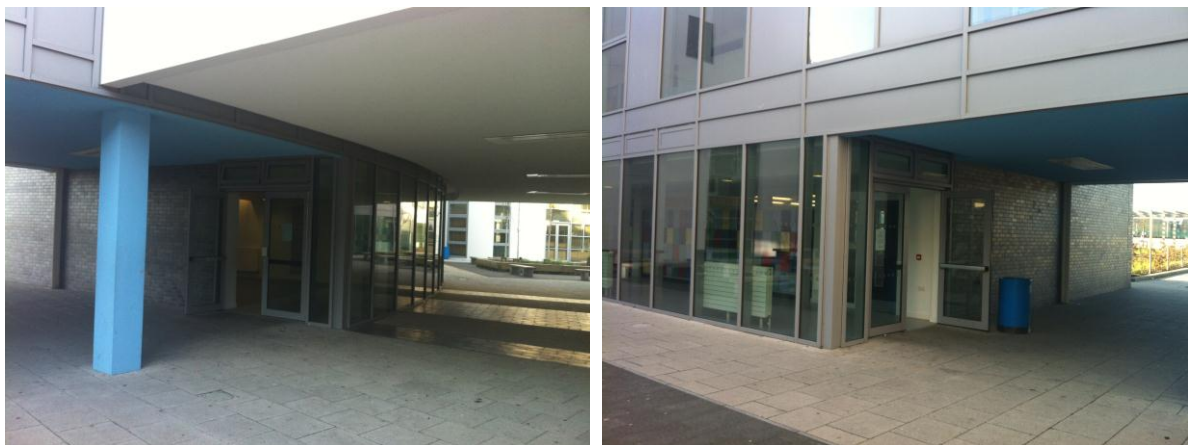
Figure 7.4: Ground level circulation doors open at both corridor ends in winter
