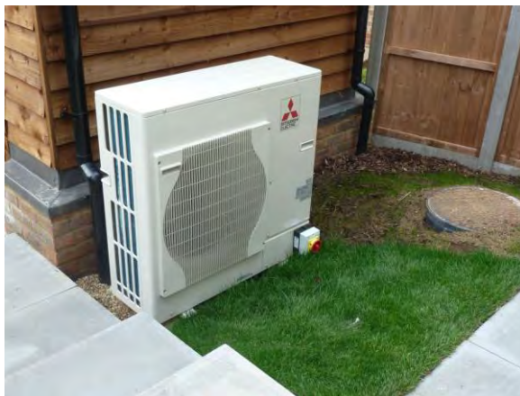
Figure 12 Air source heat pump located near the bicycle shed in the rear garden
