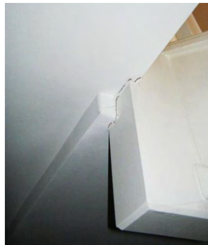
Figure 7 House 2: additional plasterboard soffits used to cover a construction flaw in the staircase
