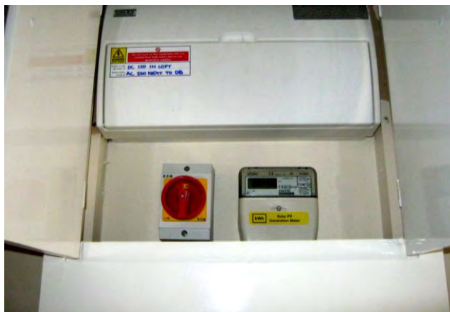
Figure 16 Solar PV generation meter
