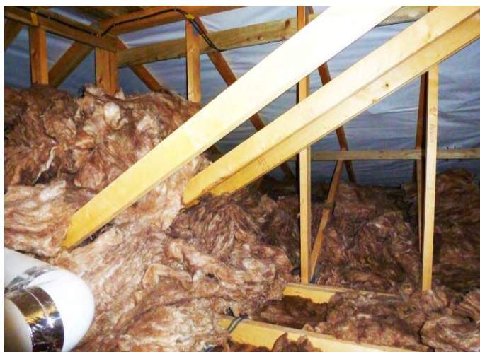
Figure 47 Roof insulation is not distributed well resulting in insulation gaps.
