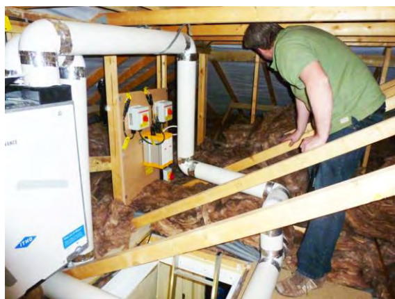
Figure 99 MVHR unit in loft space
