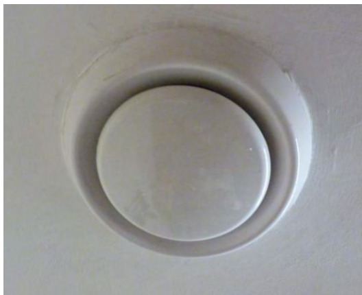
Figure 20 Extract ventilators in the kitchen
