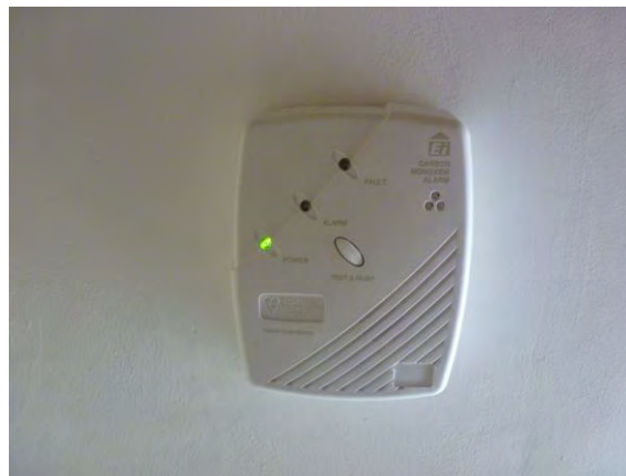
Figure 21 Carbon monoxide alarm
