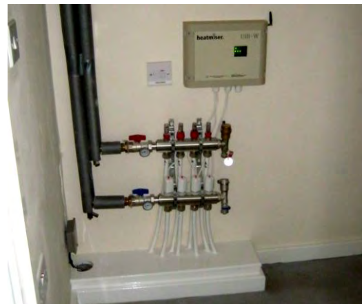
Figure 17 Control system for under floor pipework
