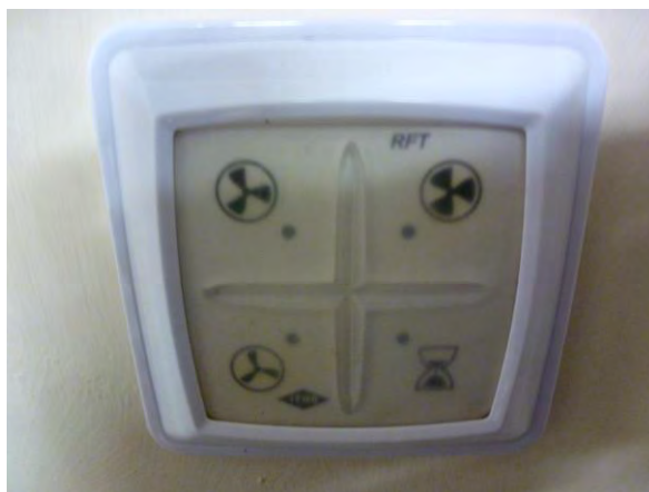
Figure 18 MVHR Boost control: Top RHS is for boosting the ventilation, Bottom LHS is for normal operation, Bottom RHS is for fixed time-period boosts
