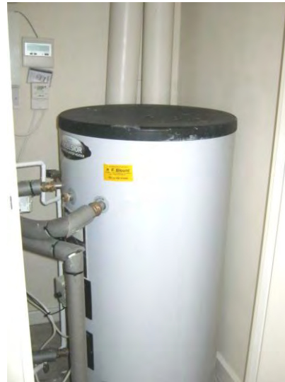
Figure 15 Hot water tank with immersion heater
