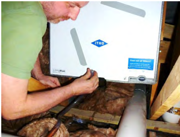
Figure 101 Condensation pipe not draining
