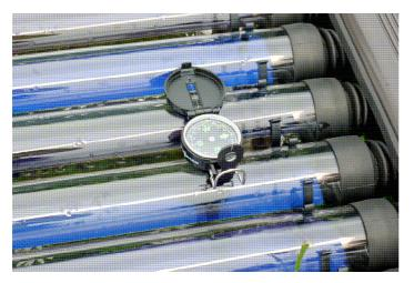
Solar thermal tubes were installed north-south instead of east-west, and a third of them were installed upside-down.
