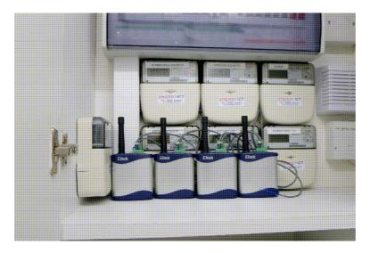
Electrical sub-meters were fitted with wireless transmitters to connect them to Eltek's datalogger.
