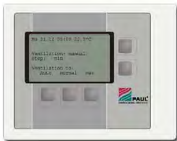
Figure 2-7. Ventilation control installed in the living room
