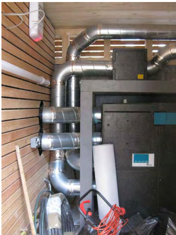
Figure 2-6. Heat Recovery Ventilation unit (BEFORE DUCTWORK WAS INSULATED) inside the frost-protected unit in the external bike shed.
