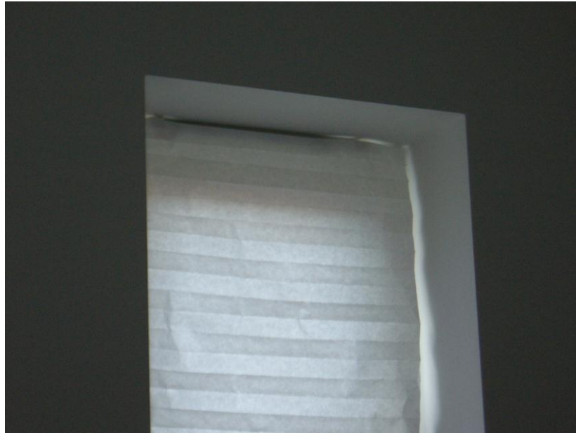
Figure 6 - Paper blind installed on the window led to the trickle vent being blocked
