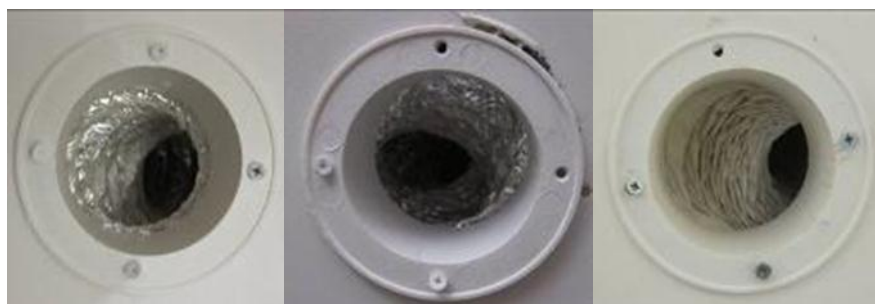
Figure 5 - Extract terminals with diffusers removed showing constrictions in flexible ducting
