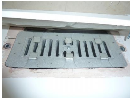
Figure 10 Adjustable grille on supply air valve.
