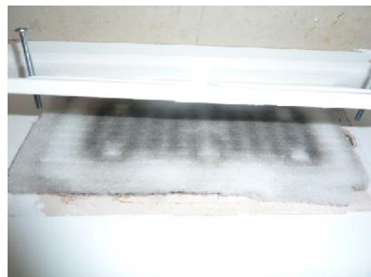
Figure 11 MVHR supply air valve and filter.
