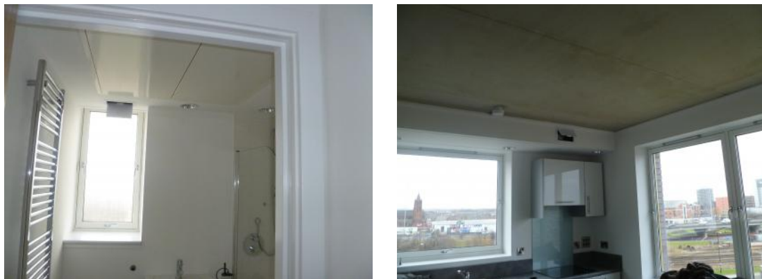
Figure 13 Extract air valve access hatch in the bathroom and living/kitchen area.
