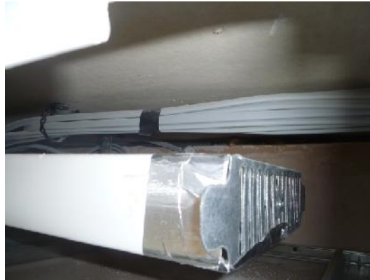
Figure 12 Grille taped to the end of the extract ductwork above the kitchen cupboards.
