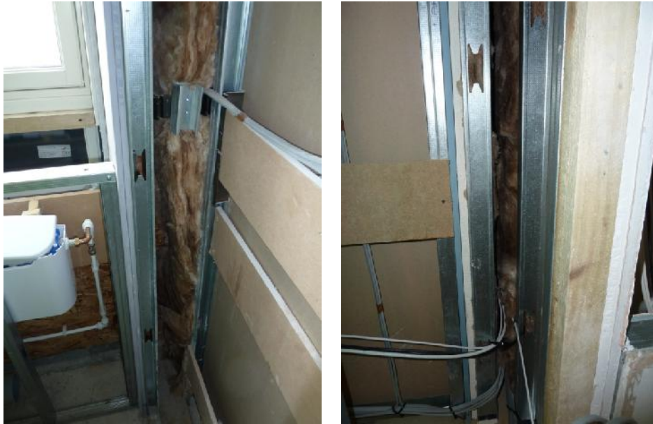
Figure 4 Insulation bridging across party wall.
