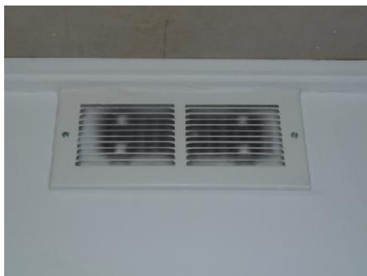
Figure 11 MVHR supply air valve and filter.
