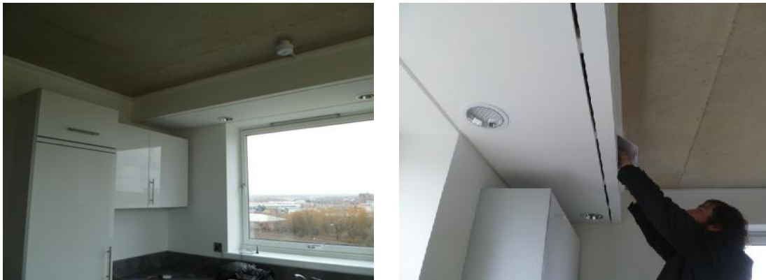
Figure 7 Extract slot above the external window in the bathroom and above the cupboards in the kitchen.
