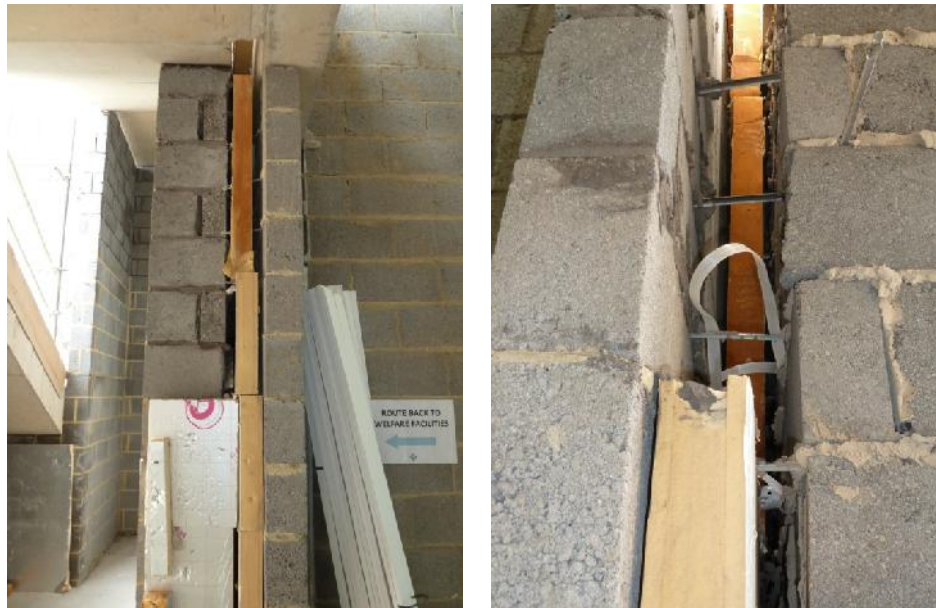
Figure 6 Partial fill insulation not securely retained at ground floor.
