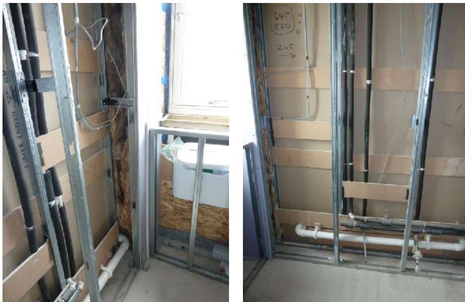
Figure 5 Services installed within party wall.
