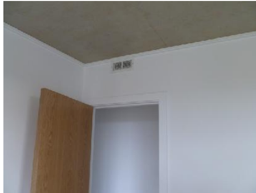
Figure 9 Supply air valve located above the door in the living room/kitchen.
