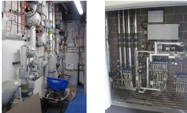
Figure 10 (Left) Low temperature hot water pipes in Ground Floor plant room. (Right) Low temperature hot water pipes in Riser A.
