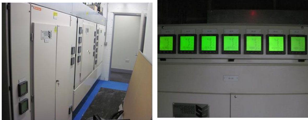
Figure 16 Left: The sub-metering arrangement in Switchroom. Right: DB/LIB1 sub-metering in Ground Floor Riser A.
