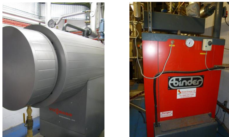
Figure 9 (Left) Gas boiler located in Ground Floor plant room. (Right) Biomass boiler located in Ground Floor plant room.
