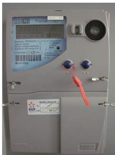
Figure 14 Entity PRI electricity meter located in the ground floor Switchroom.
