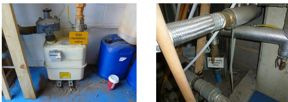
Figure 7 (Left) Actaris Itron gas pulsed output meter located in the Ground Floor plant room. (Right) Main water service isolation valve in Ground Floor plant room.
