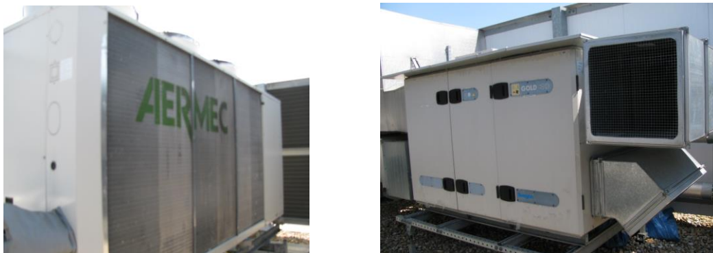
Figure 12 Air cooled liquid chiller located on the roof.
