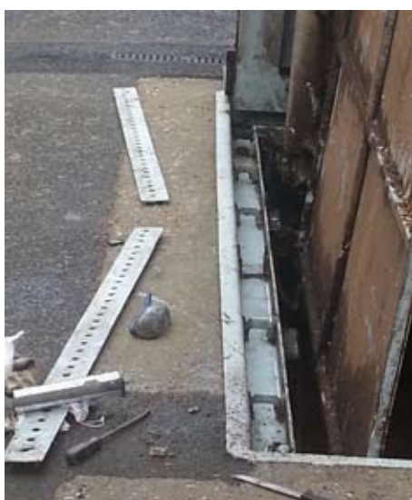
Figure 7.2: Channel hole widening in February 2012 showing the new drainage channel from measure 4 (top) and the debris covers from measure 1.
