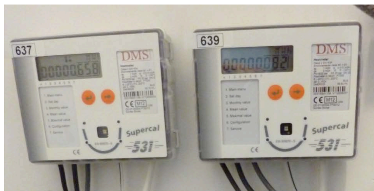
Figure 13 Installed Heat meters in MWh resolution
