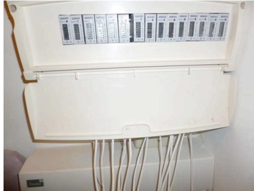
Figure 15 Unlabelled wiring
