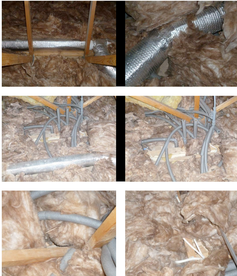
Figure 6 Discontinuities in the insulation layer in the loft space.
