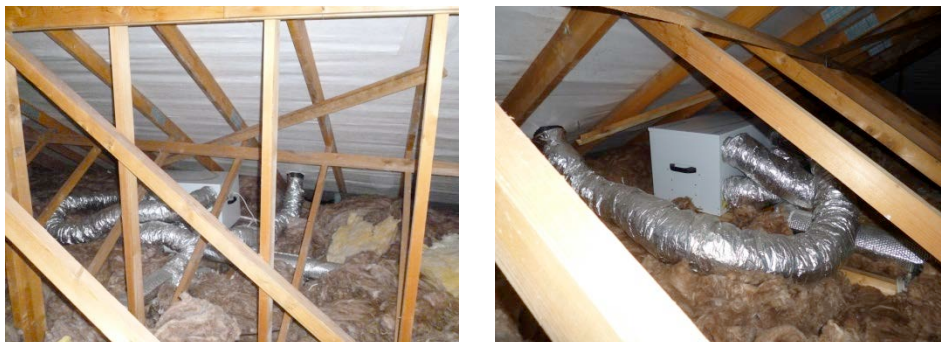
Figure 5 Location of the MVHR unit within the loft space.
