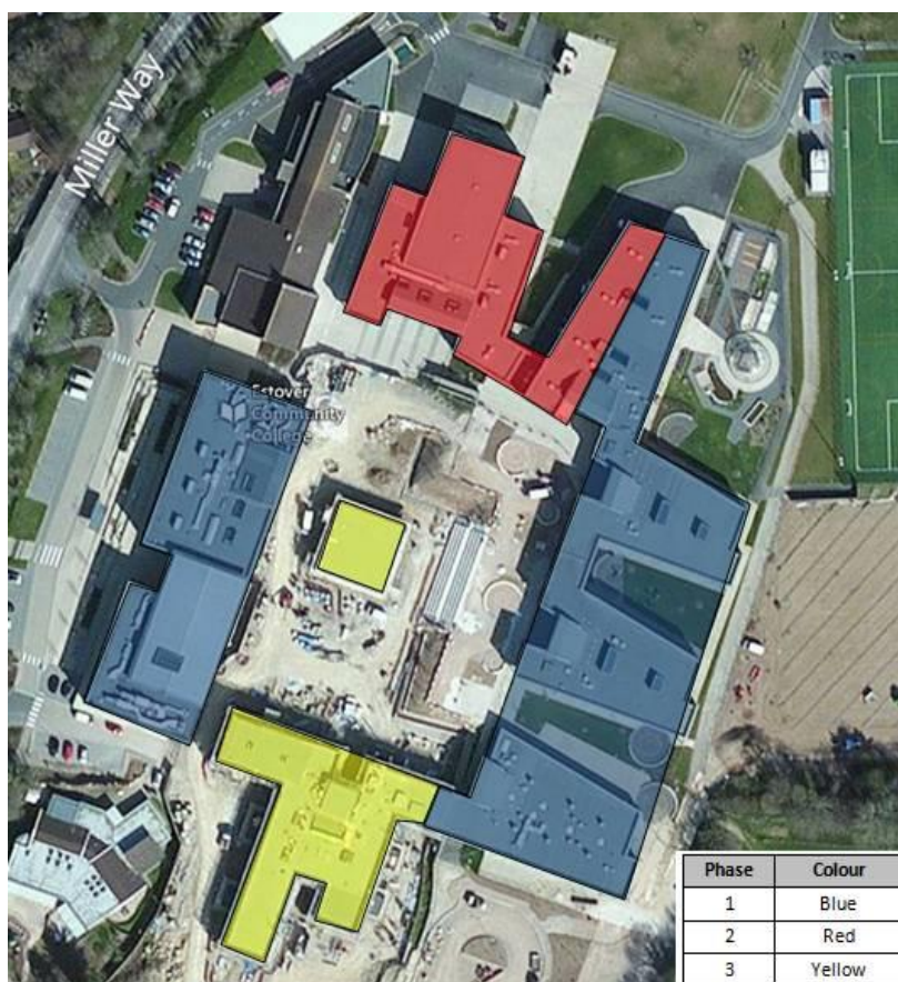
Figure 2.1. Aerial photograph showing the construction phasing plan.
