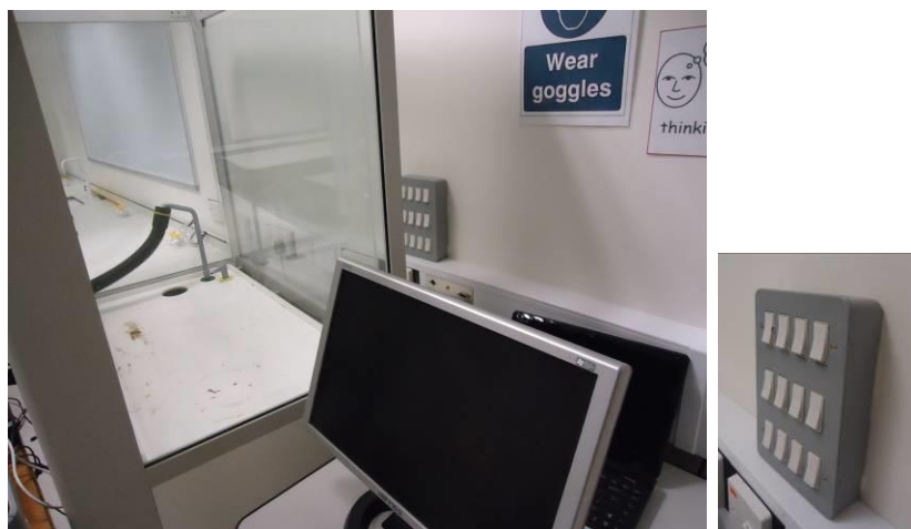
Figure 10.37. Lighting control in Science Opportunity Centre obscured by fume cupboard and PC, note there are no labels to inform the user which lights the control is for.
