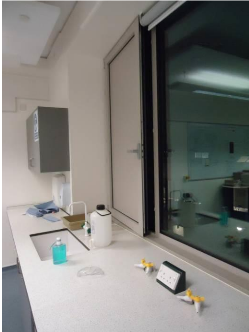
Figure 7.7. Night vents left open overnight in winter.
