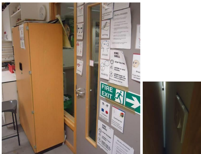
Figure 10.36. Art room L210 Cade North, note the light switch obscured behind a cupboard
