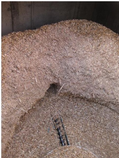
Figure 7.3. Photograph showing build up of woodchip in corners of storage pit.
