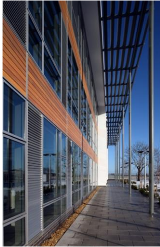
Figure 1.1: South East Facade with Solar Shading
