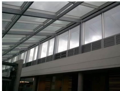
Figure 3.5 Natural Ventilation
