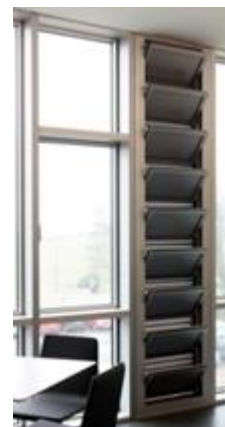
Figure 1.5: Automatic Louvres
