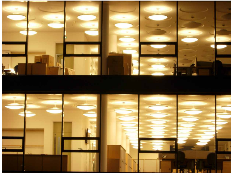
Figure 29 Ground floor open plan office indicating density and patterns on internal electric lighting
