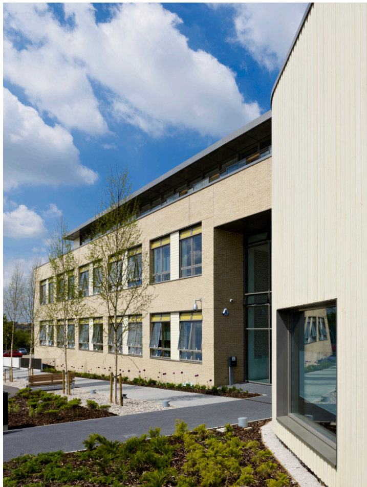
Figure 8 View of entrance with timber frame and brick finishes
