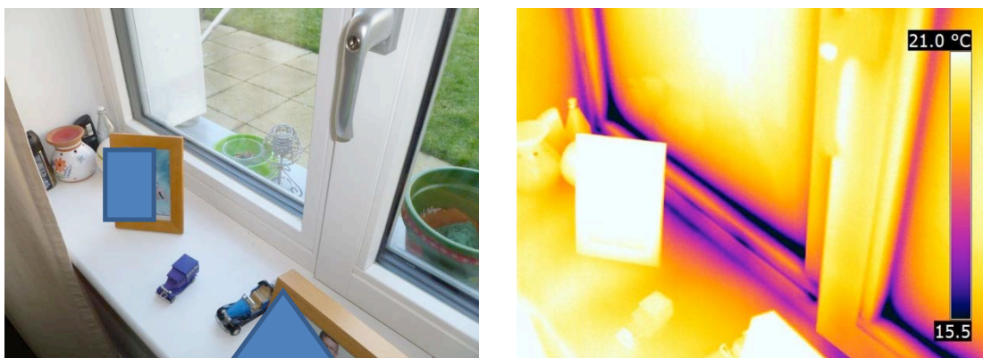
Figure 10 Leakage between the joints in the frame of the window in the master bedroom.
