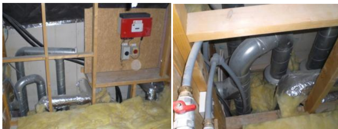
Figure 5 NIBE cupboard. Gaps in insulation and air leakage paths.
