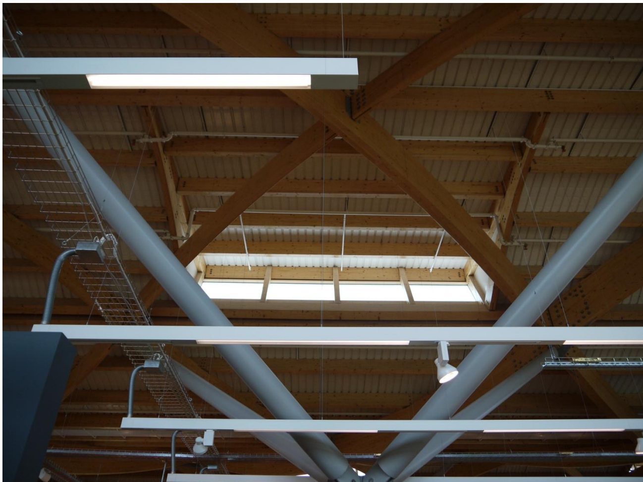
Figure 60 – Internal roof showing steel support tree, glulam roof frame, track lighting and north light
