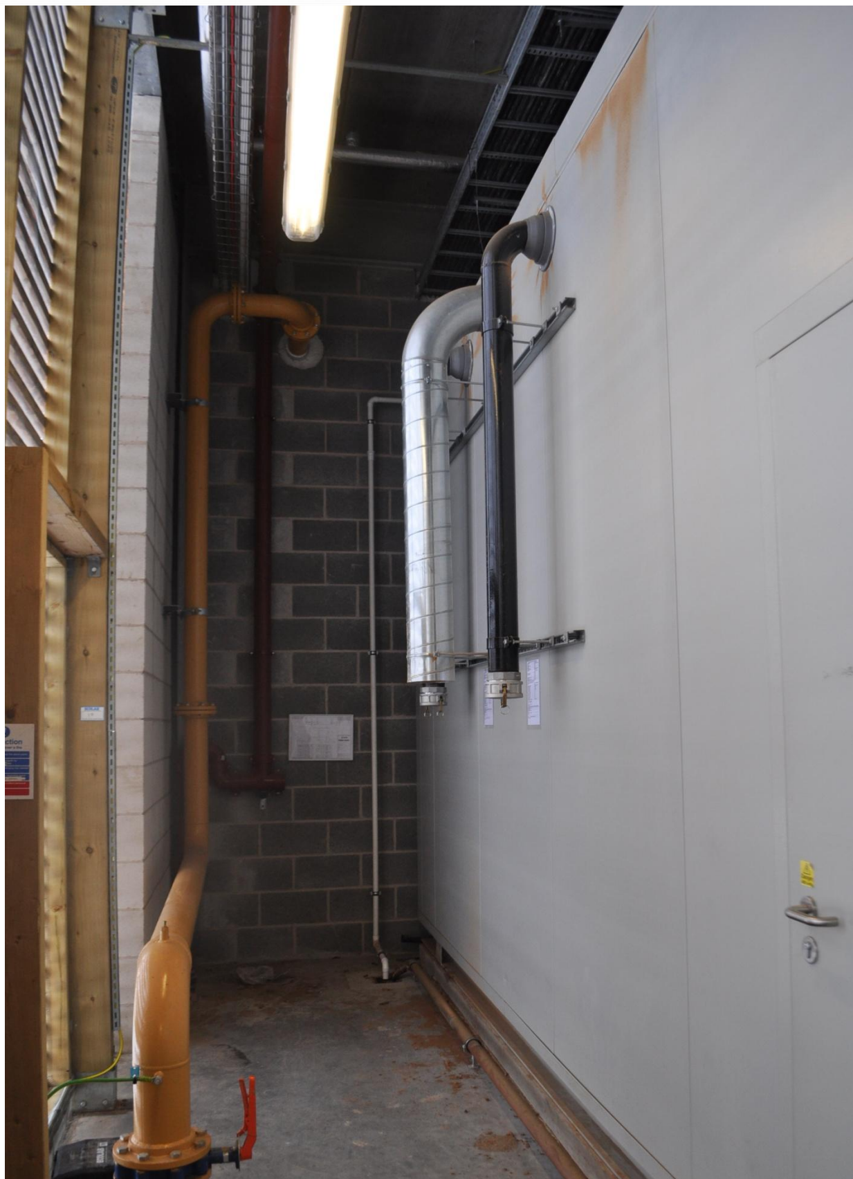
Figure 64 – Biomass boiler wood pellet delivery chute
