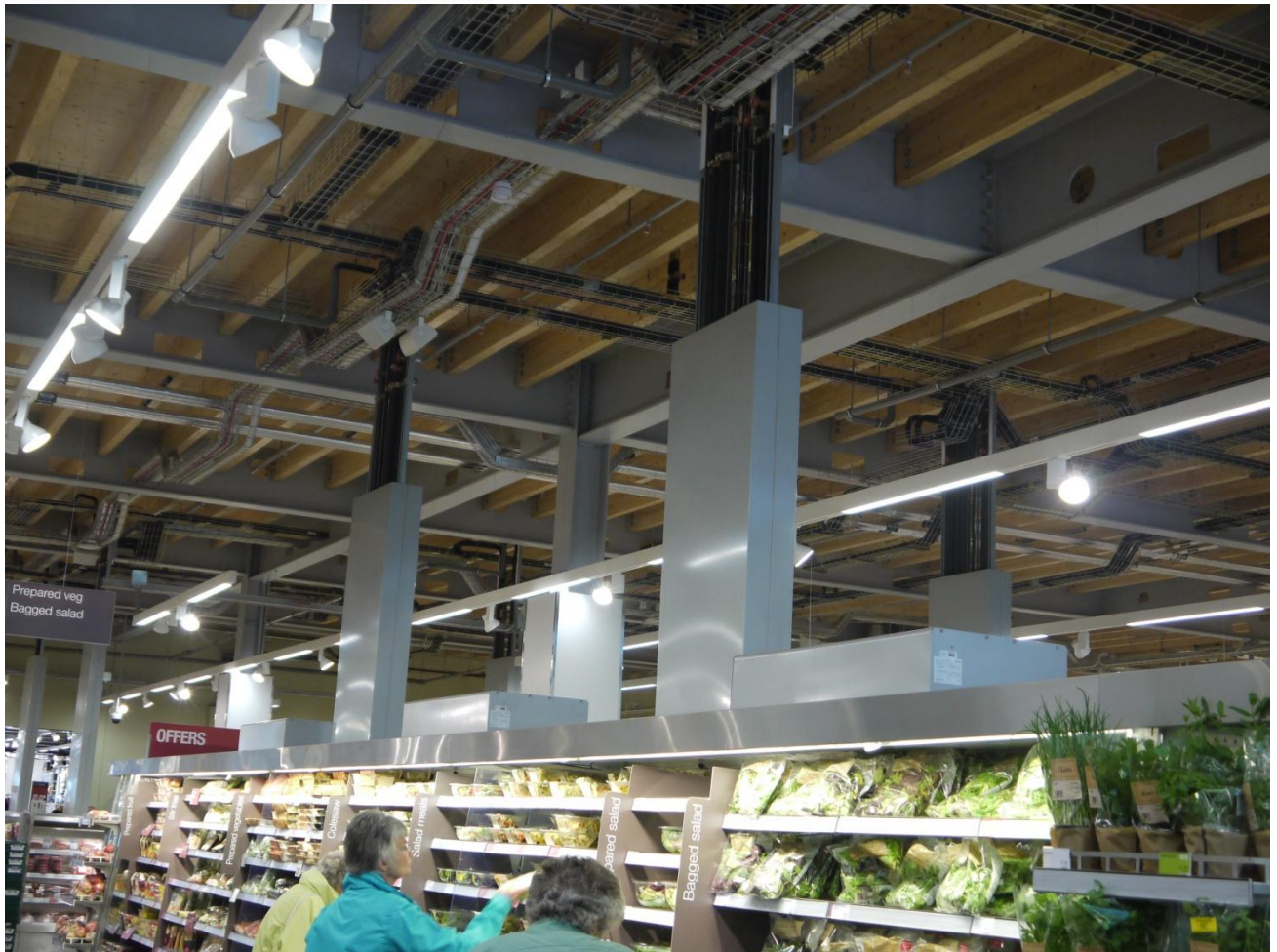
Figure 62 – Chilled food cabinets with top entry CO 2 connections
