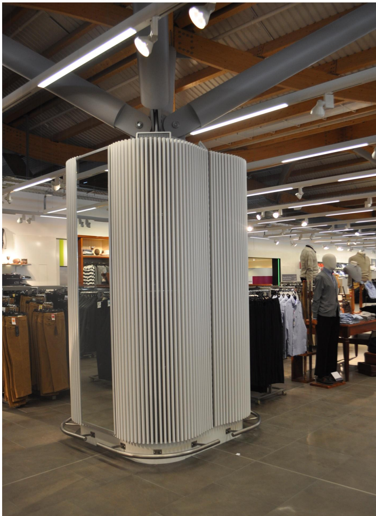
Figure 59 – Displacement ventilation column
