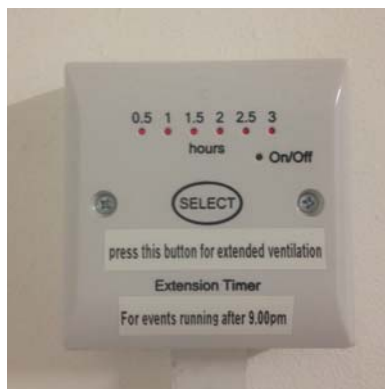
Figure 3-6 Ventilation extension timer (basement, main staircase hall)
