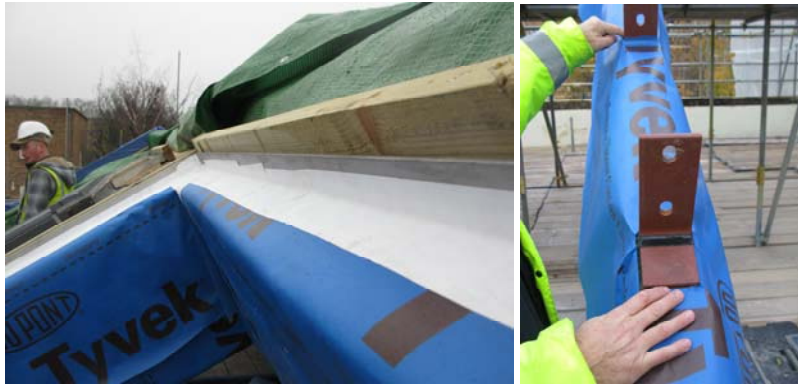
Figure 2-13 Airtightness tapes around windows (previous page) and thinking ahead with membranes fitted to rooflights and trusses in readiness for later connection to the main membranes.
