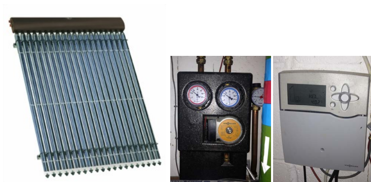
Figure 3-16 Solar thermal panel, pump and control display
