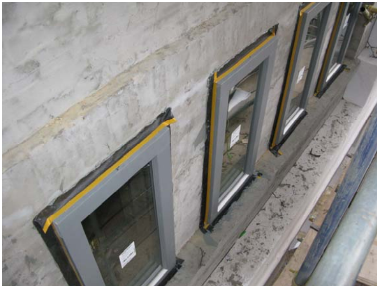
Figure 2-12 Location of windows into wall build-up
