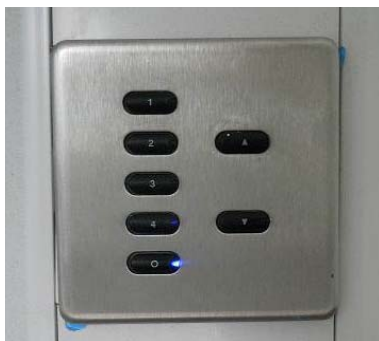
Figure 3-18 Light switches with controls for dimming or selecting pre-set light levels
