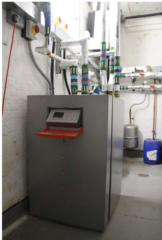
Figure 3-8 Ground source heat pump (GSHP)
