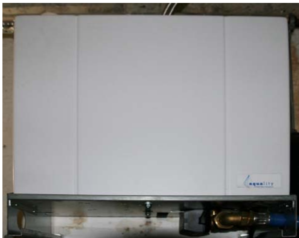
Figure 5-9 Aqualite rainwater harvesting pump
