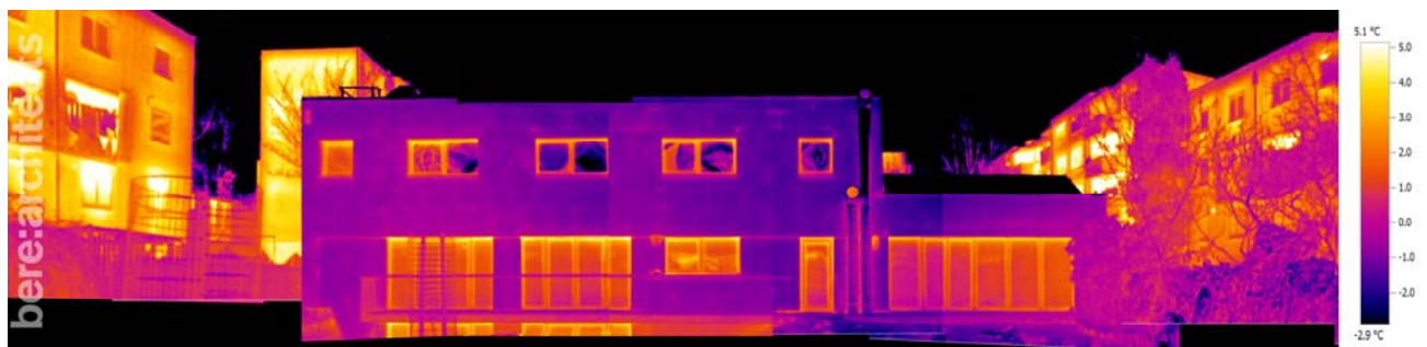
Figure 5-1 Mildmay Centre – thermographic image of the south elevation and near-by estate with high heat losses (note: windows reflecting heat from uninsulated building behind camera)
