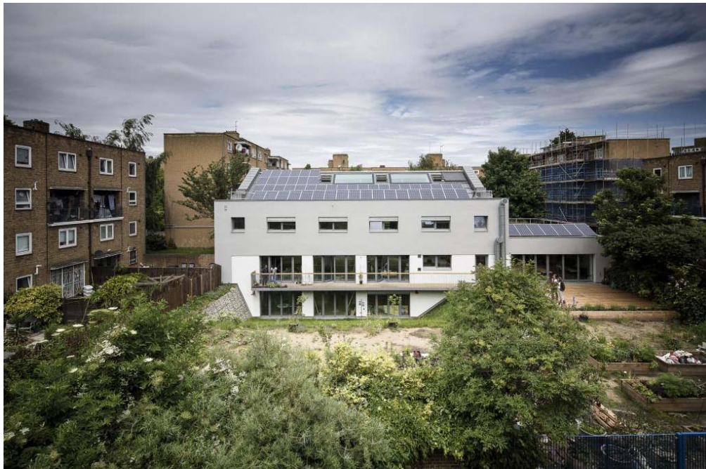
Figure 3-14 Mildmay Centre - photovoltaics arrays (on the main zinc roof and on the ground floor extension)
