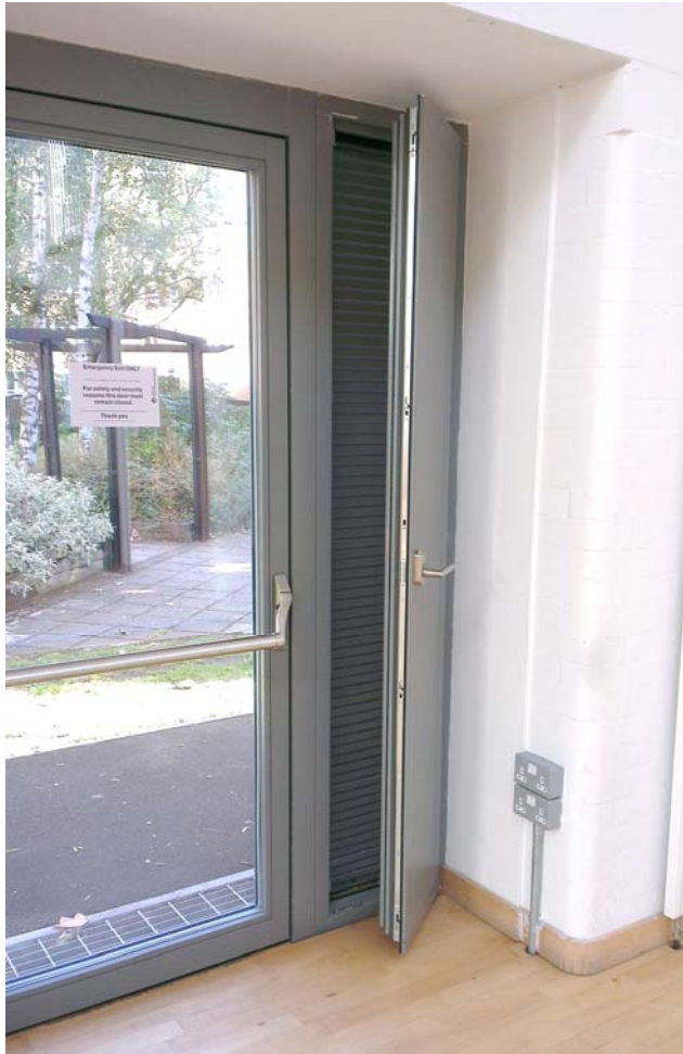
Figure 5-5 Ventilation grille (main hall)
