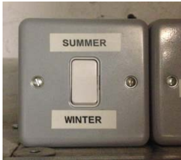
Figure 3-3 Ventilation unit – summer/winter strategy switch (plant room)
