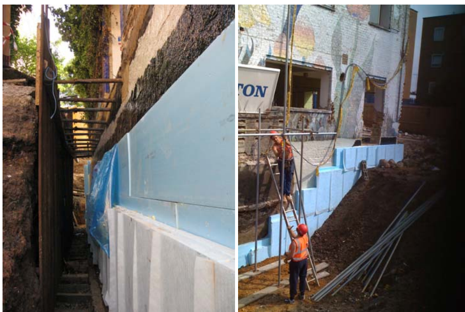
Figure 2-5 Insulation at basement level
