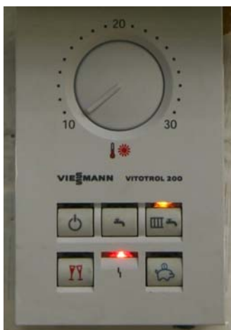
Figure 3-10 Thermostat and DHW & heating controls (main hall)
