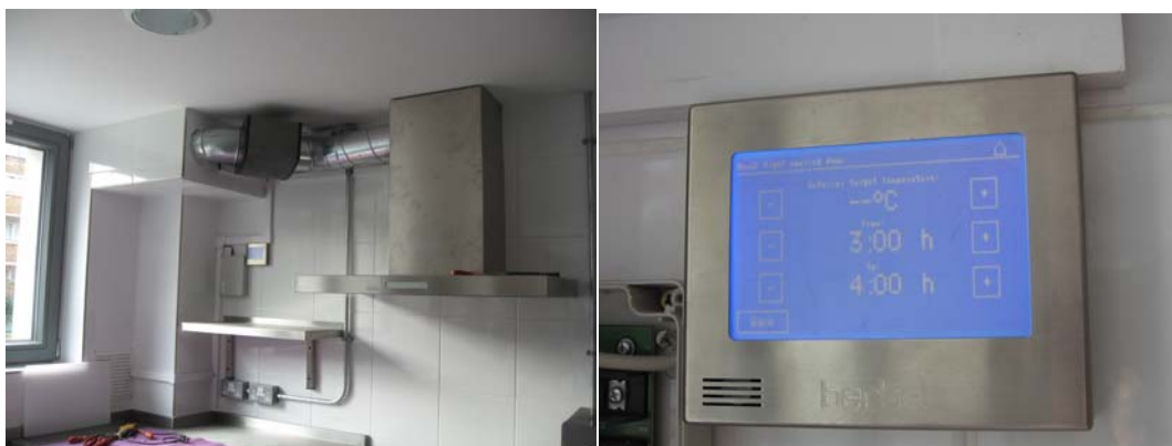
Figure 3-7 Kitchen hood, filter and controls display
