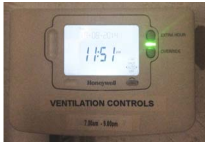
Figure 3-5 Ventilation timer control unit (plant room)
