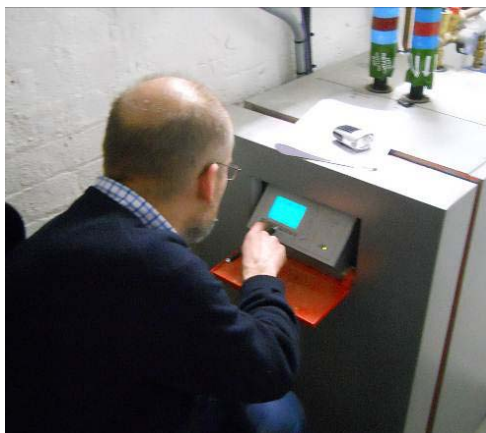
Figure 3-11 GSHP control display
