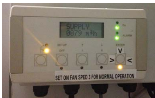
Figure 3-2 Ventilation unit – controls display (plant room)
