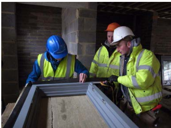
Figure 4-1 Window airtightness taping – training on site
