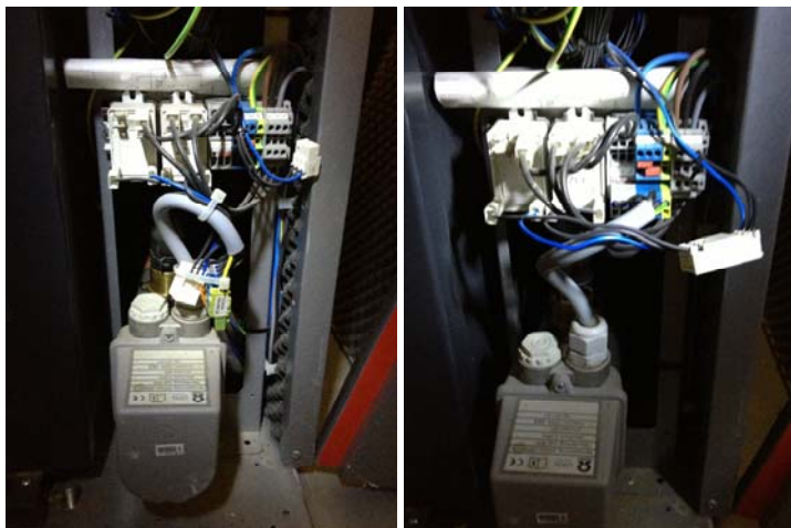
Figure 3-12 The GSHP direct heater as found in May 2013 (left), and after it was connected (right)
