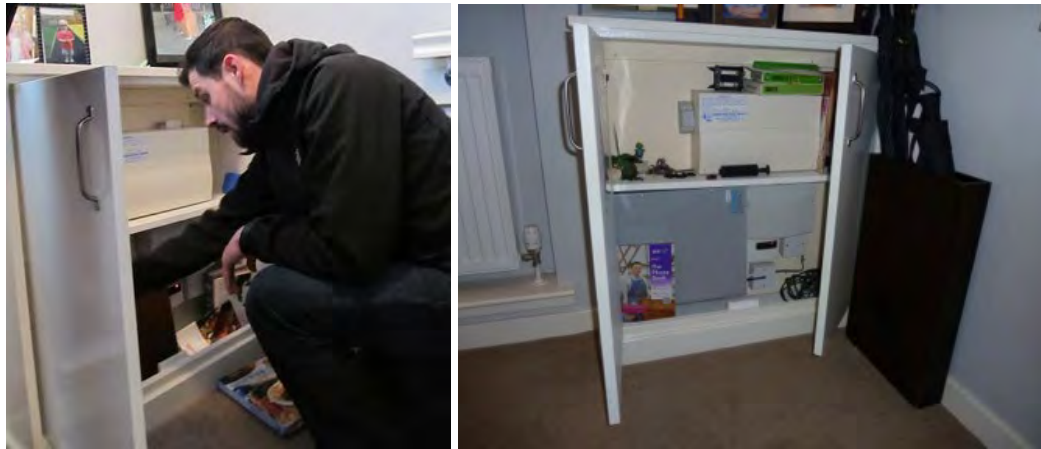
Figure 55: Installation of T-Mac unit in meter cupboard.
