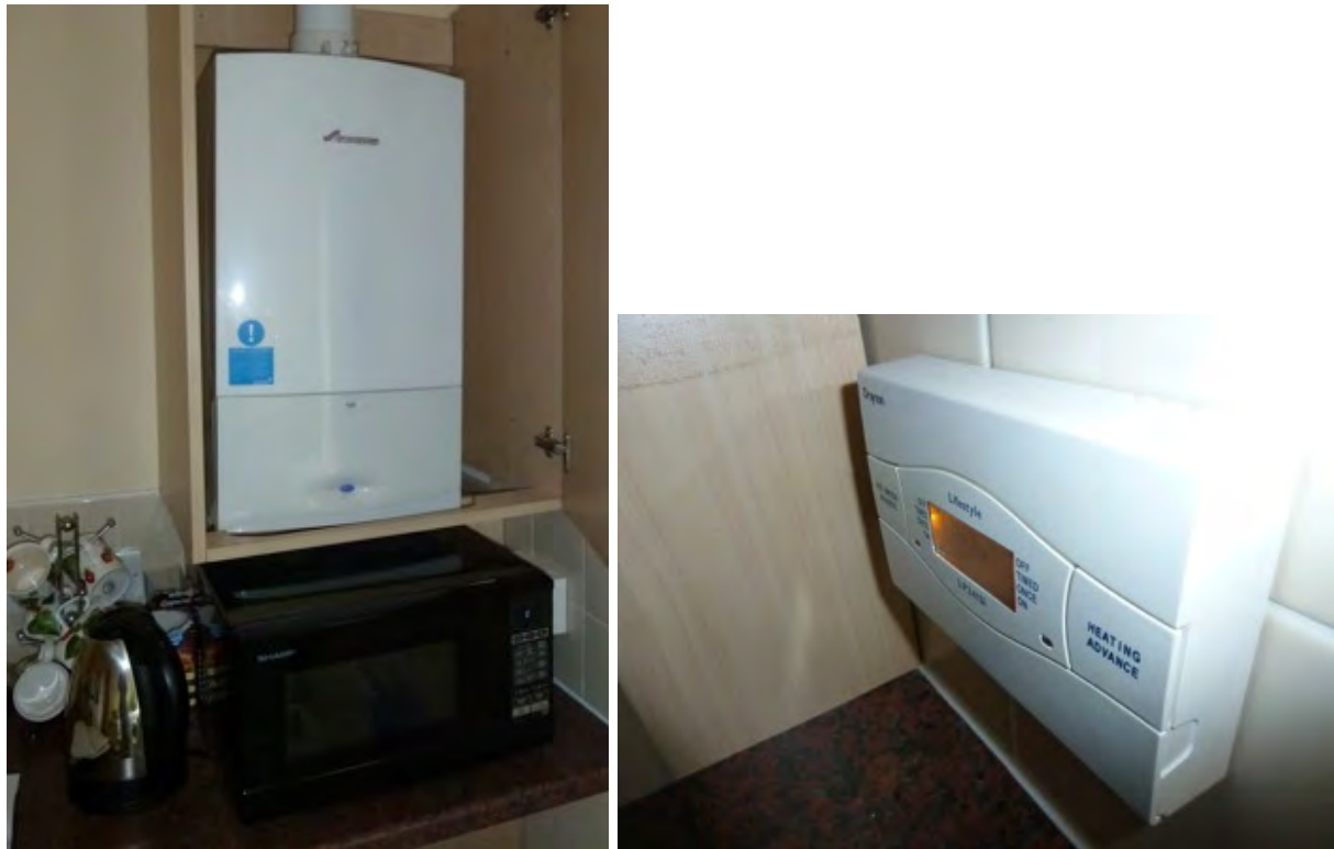
Figure 49: Boiler located in the kitchen (left); programmer located below the boiler (right) - note access to programmer (blocked by the location of Microwave oven).
