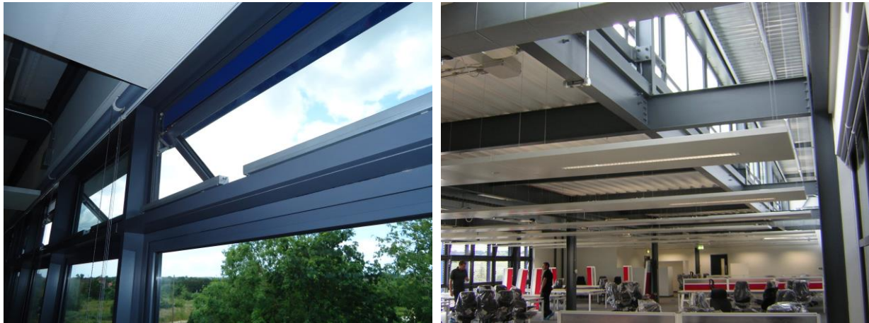
Figure 7.9: (Left) Automated windows in a first floor office area and (right) East Office.
