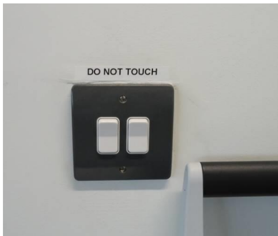
Figure 7.10: Manual override for automated windows. Note the text discouraging occupants from using the control and the lack of explanatory labelling explaining.
