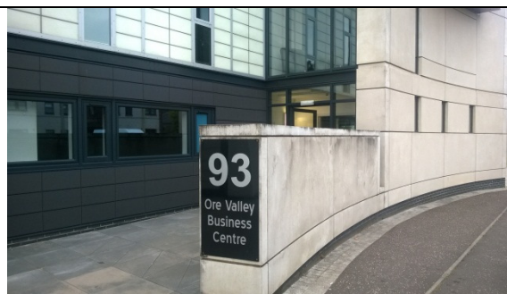
Figure 7: Wall at the entrance area in front of the ground floor open plan office, forming a sound buffer.
