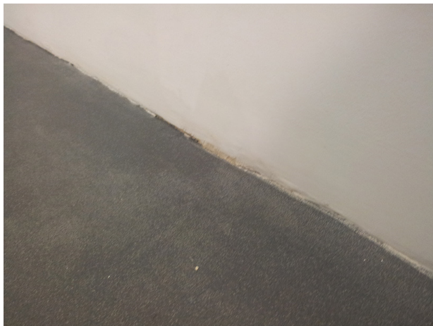
Photograph 4 rear entrance corridor. Image indicates area of floor where ponding occurred.
