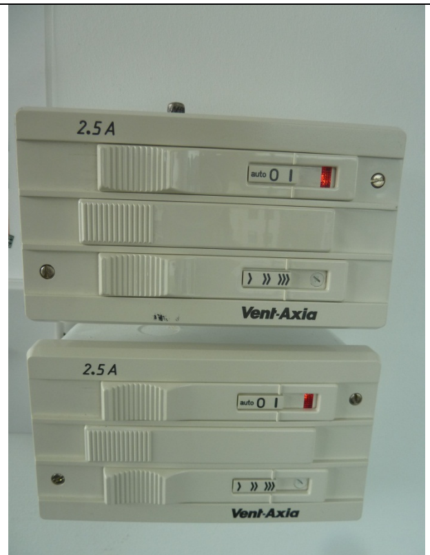
Figure 13: Extract fan controls shown operating at high speed.
