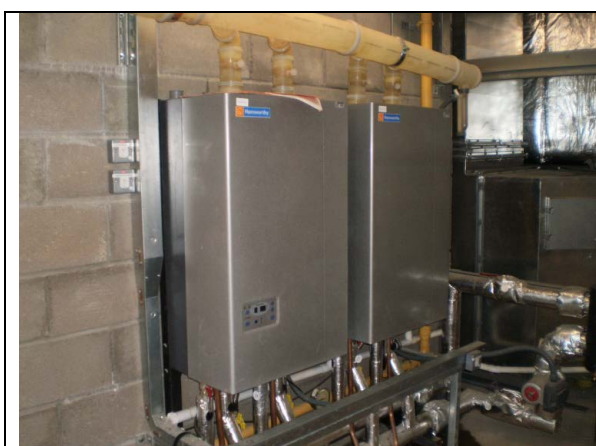
80kW boilers serving both systems
