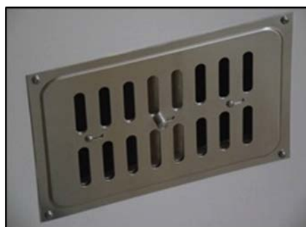
Picture 22: Hit-and-Miss vent closed for duration of testing
