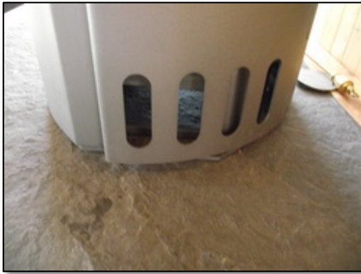
Picture 28: Substantial leakage through base of wood-burning stove in living room
