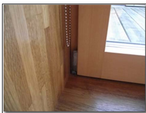
Picture 27: Substantial low level leakage at hinge side of balcony doors in two bedrooms, Doors DF.02 & DF.03
