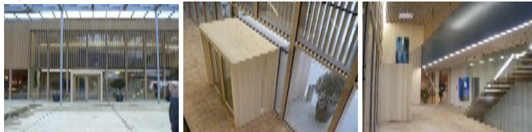
Picture 11: Ludesch Town Centre – constructed from Brettstapel
