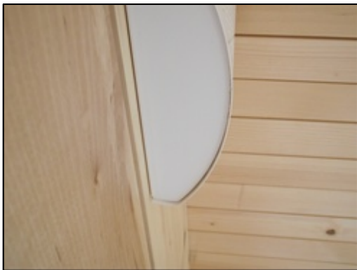
Picture 32: Leakage along back edge of ventilation terminal
