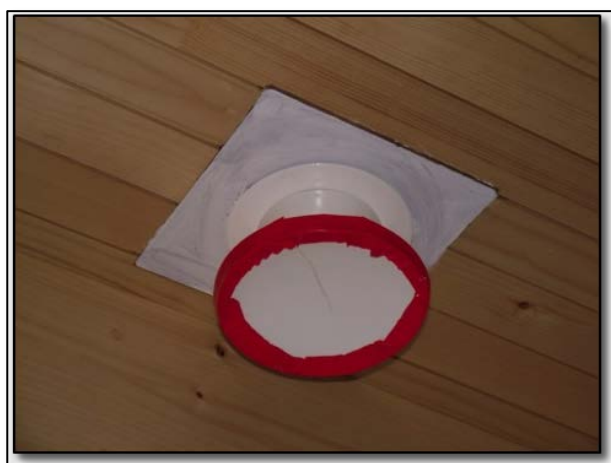
Picture 19: Supply terminal in lounge temporarily sealed for duration of testing
