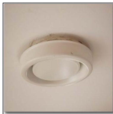
Picture 25: Leakage between ventilation terminals & adjacent plaster board ceilings and walls
