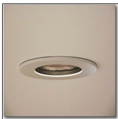
Picture 24: Leakage between spotlight fittings and adjacent plasterboard ceiling
