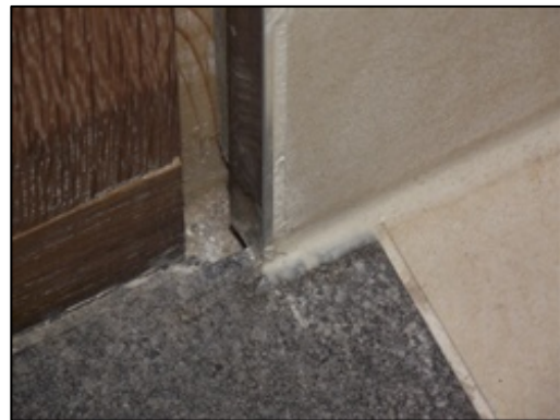
Picture 33: Leakage at edge of tiling in downstairs bathroom. Some leakage at side of the window
