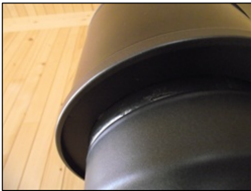
Picture 30: Leakage fire cement ineffective at junction between wood-burning stove & chimney
