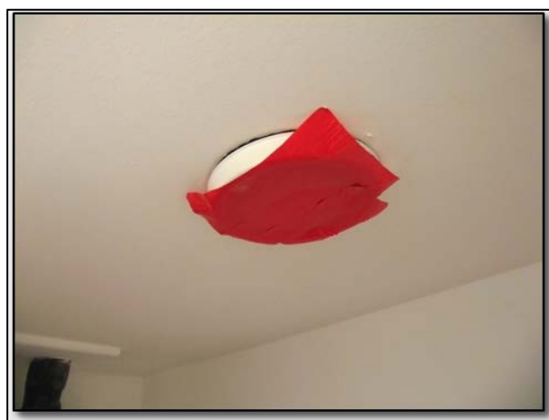
Picture 20: Extract terminal in bathroom temporarily sealed for duration of testing
