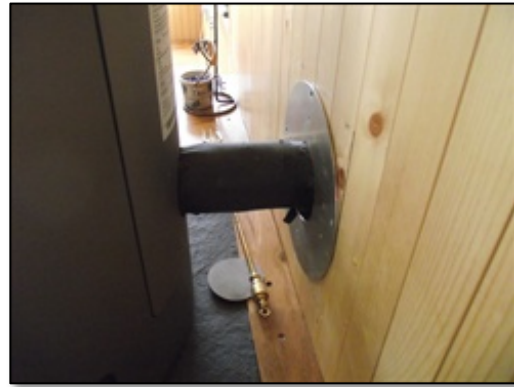
Picture 29: Leakage around external air supply to rear of wood-burning stove in living room
