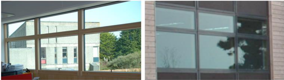
Figure 7 Windows, interior and exterior view
