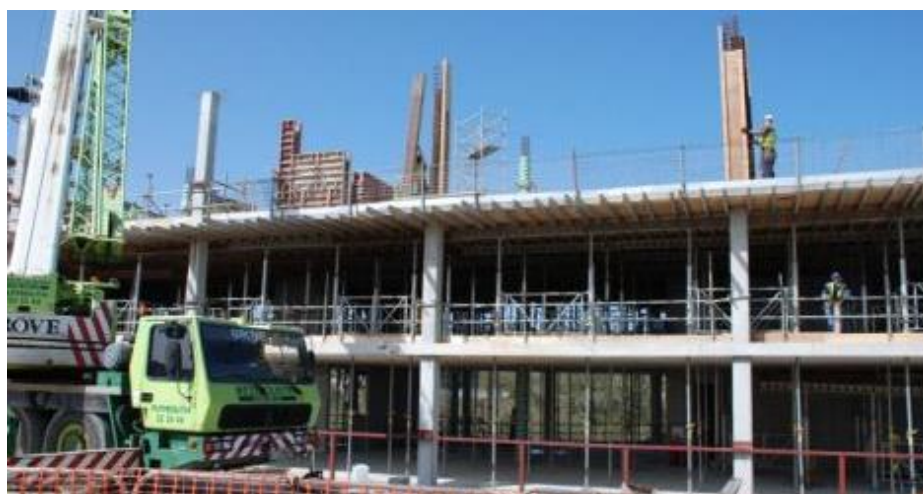
Figure 13 Construction photo showing the concrete frame under construction
