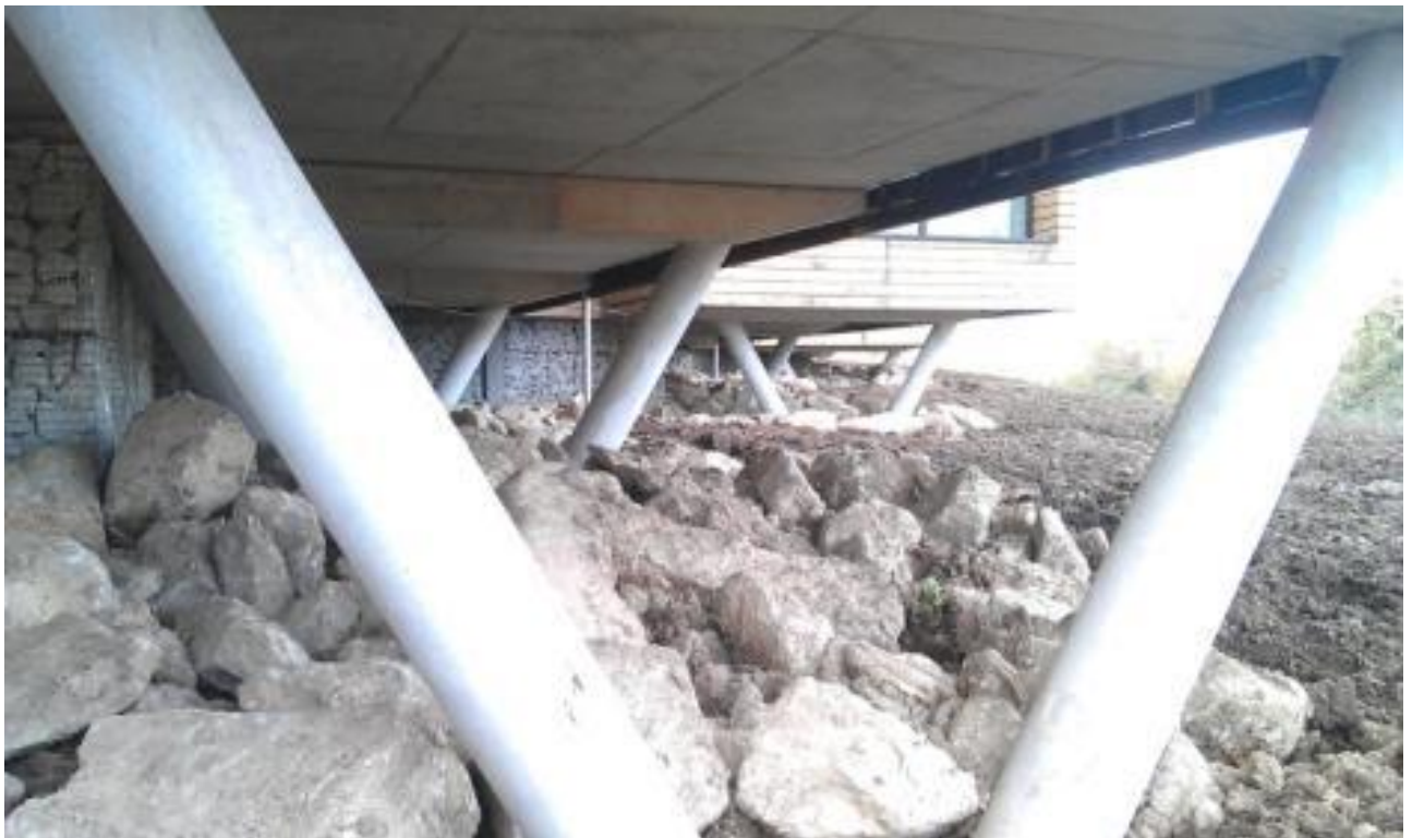
Figure 14 Suspended concrete slab at the north-east corner of the building
