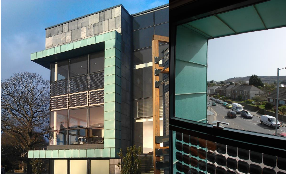
Figure 24 Solar PVs incorporated into curtain wall
