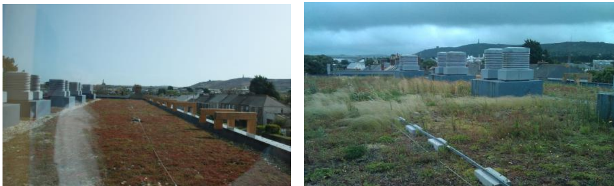
Figure 8 Extensive sedum roof and wind-catcher vents, six months apart
