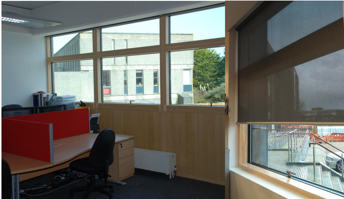
Figure 21 window controls at IC and brise soleil
