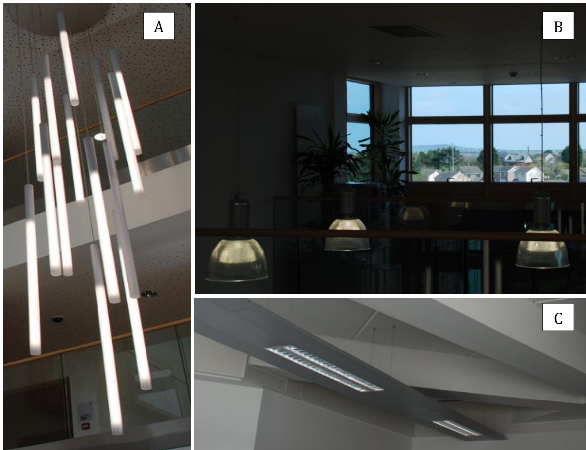
Figure 22 A Feature lighting in atrium, B Suspended lighting in atrium, C Fluorescent strips
