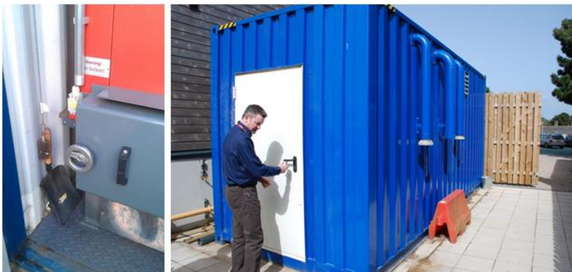
Figure 18 Tools required for manual de-ashing and the containerised woodchip store and boiler house
