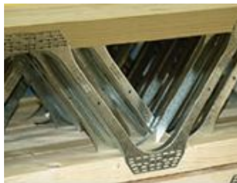
Figure 2.8; Installed open web composite beam
