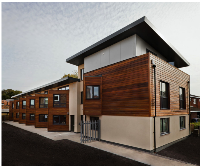
Figure 1 A picture of the northerly & west elevation of the development shortly after completion
