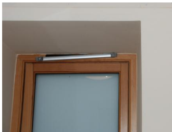
Figure 6:10: Broken trickle vent in bathroom, dwelling D2.
