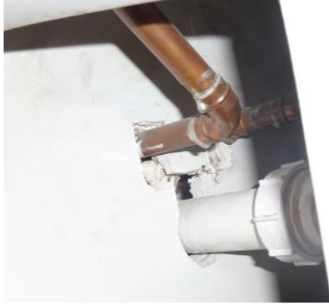
Figure 6:5: Uninsulated pipework serving bathroom wash basin. Note inadequate sealing around pipe penetrations and also excess solder flux on pipe elbows, indicating poor workmanship.
