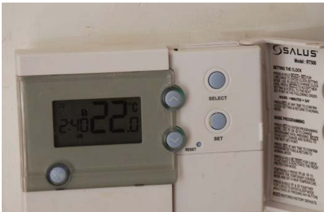
Figure 8:9: Underfloor heating programmer with date and time incorrectly set Dwelling A1.
