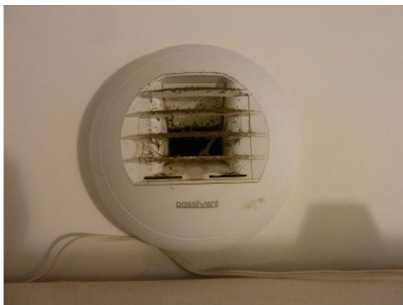
Figure 6:7: Soiled extract inlet grille in kitchen, dwelling C1.
