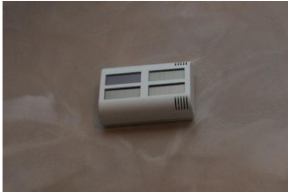
Figure 7:1: Combined temperature, relative humidity and CO 2 sensor.
