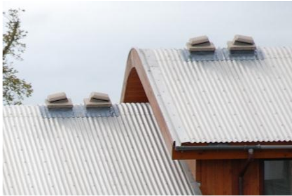
Figure 6:3: Outlets of passive stack ventilation systems.
