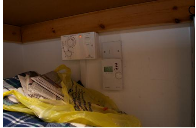
Figure 6:6: Heating programmer at rear of cupboard housing domestic hot water tank out of view (dwelling C1), note items stored on top of the domestic hot water tank restricting access to the control panel.
