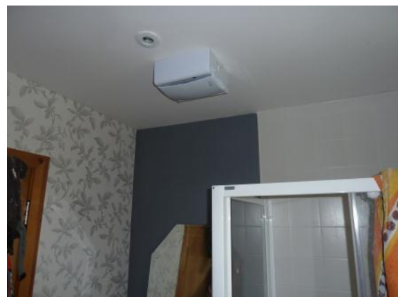
Figure 6:2: Replacement extract fan in ground floor shower room in dwelling A1.
