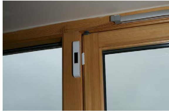
Figure 7:2: Window contact sensor.
