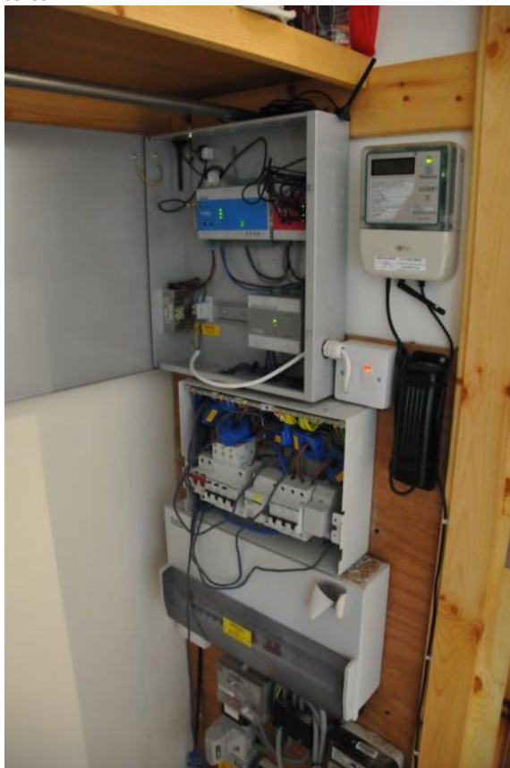
Figure 7:3: CT clamps on consumer unit (middle) and central t-mac unit (top left). Electrical Orsis meter top right of image.
