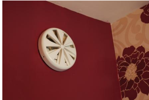
Figure 6:4: Typical inlet grilles of passive stack ventilation system, humidity activated. (WC in B2).
