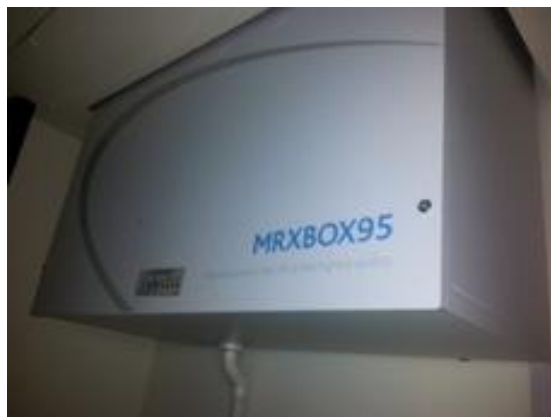
Figure 6.1: The installed MVHR unit in one of the Flats
