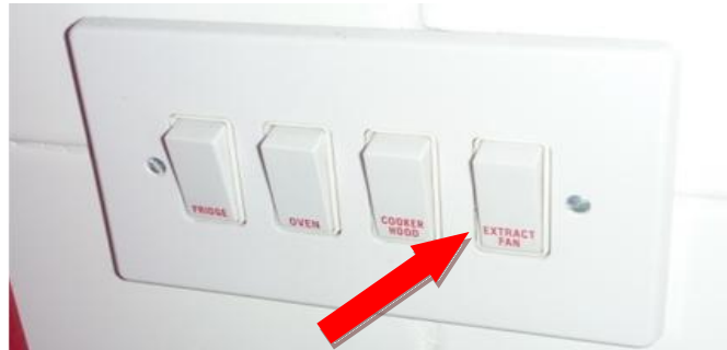
Figure 6.3: The switch gang in the kitchen where the switch for MVHR boost is located, labelled as 'extract fan'
