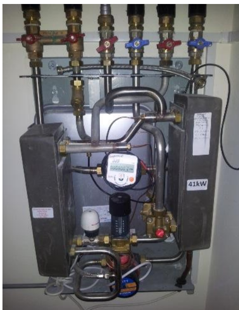
Figure 6.10 An HIU with the metal encasement removed to show the internal pipework and components.
