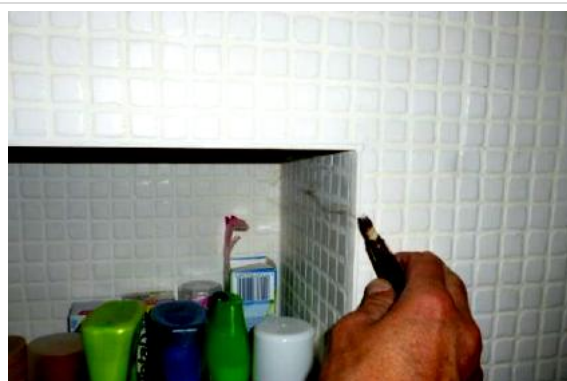
d) Penetration at sink cut out in bathroom
