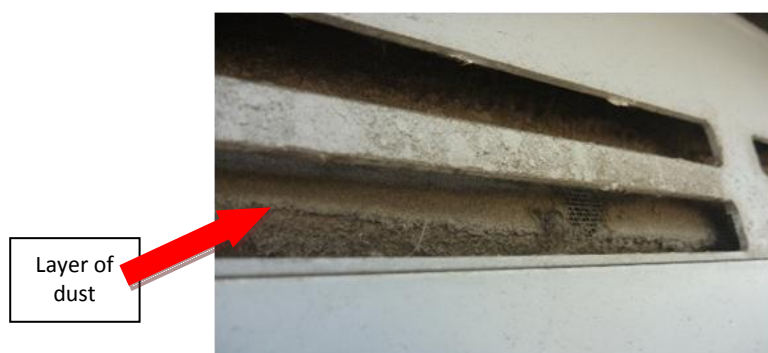
Figure 6.6: The MVHR inlet grille insect mesh heavily clogged up with dust. There is no clear way to remove the mesh for cleaning apart from via vacuum cleaning
