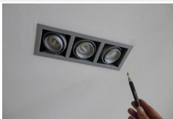
c) Air leakage around light fitting in Flat 2 living room
