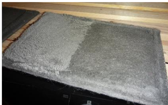
Figure 6.5: The MVHR extract side filter showing the difference between before and after cleaning, illustrating the extent of dust clogging up the MVHR at the time of the survey.
