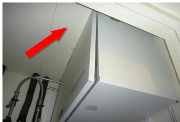
Figure 6.4: The constraints with opening the MVHR front panel due to placement of the unit part way into the false ceiling
