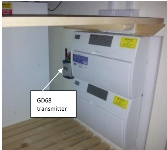
Figure 7.1: Photos of consumer units post-installation
