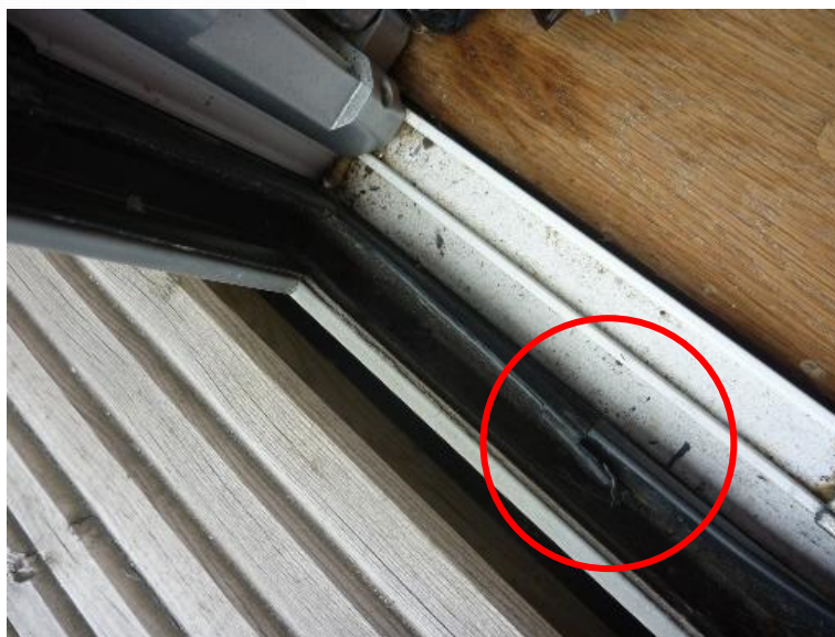
Figure 4.1: Balcony door seal, where the joints have started to fail, which would compromise the air-tightness of the property
