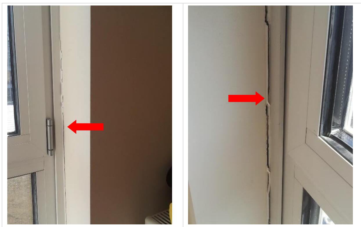
Figure 4.2: Cracks found in Flat 3 at the wall interface with the windows
