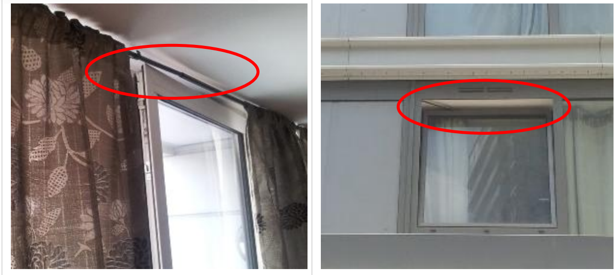
Figure 4.3: The narrow gap available between the windows/doors and the false ceiling, making the opening of fenestrations difficult and restricting ventilation
