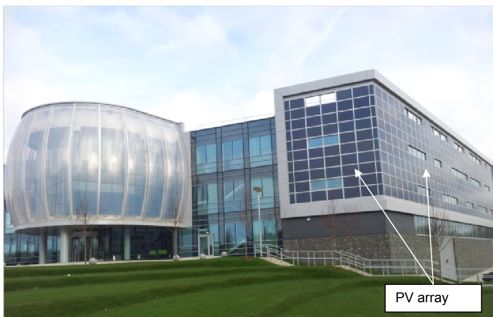
Figure 13: Photo showing PV array on South and South west facade.
