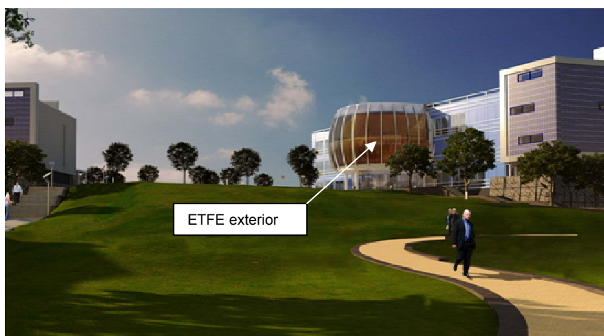
Figure 5: Photo render showing ETFE (“the bubble”) exterior around hub of Incubator building
