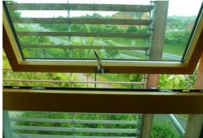
Figure 7.1 operable window – limited opening distance
