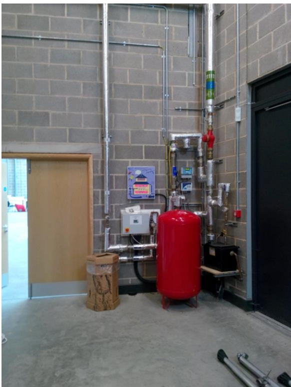
Figure 7.7 & 7.8 rainwater harvesting system and display located in the ground floor workshop store.
