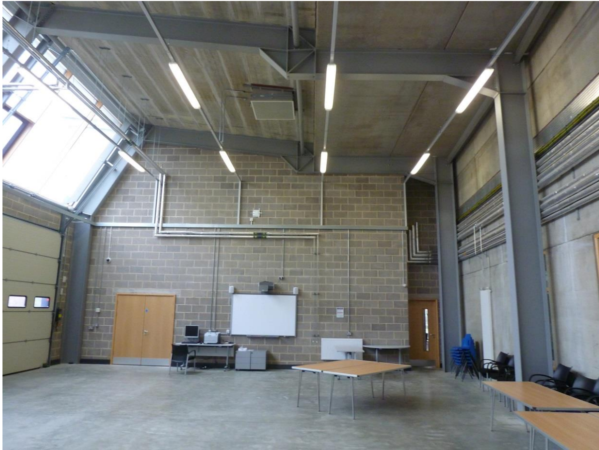
Figure 4.11 Workshop (northwest corner)
