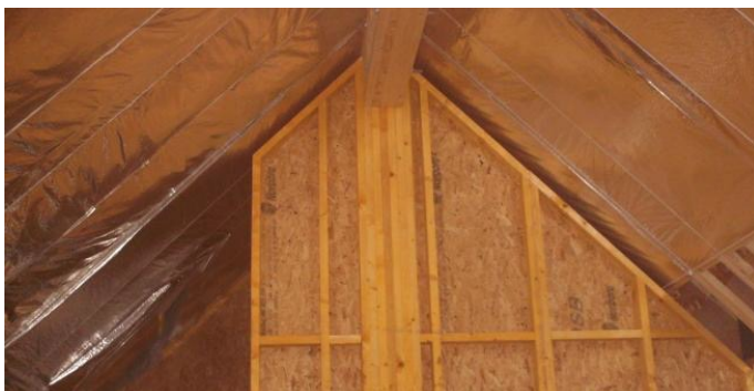
Figure 2.6: PassivWall closed panel timber system by RTC Timber Systems.
