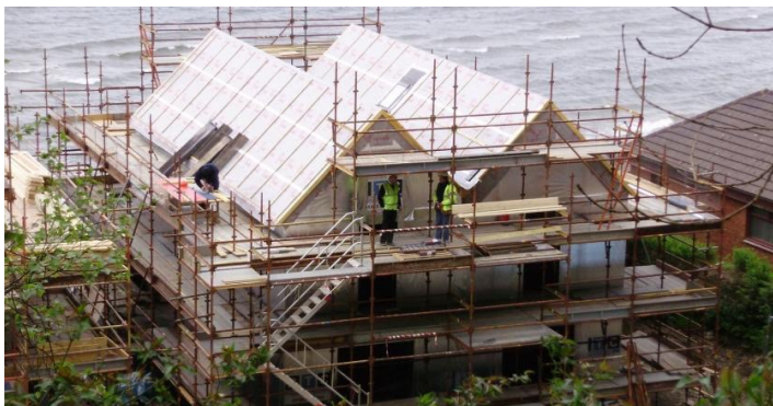
Figure 2.4: PassivHaus on the right of image has thicker layer of roof insulation (grey).
