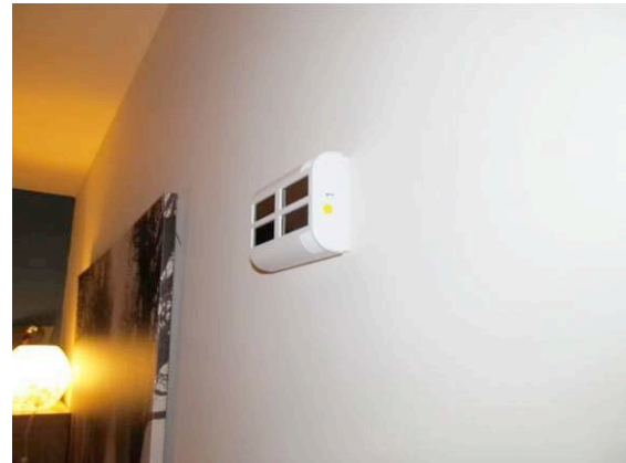
Figure 7.2: Living room: installed environmental monitoring (CO 2 , Temperature and RH%) sensor.
