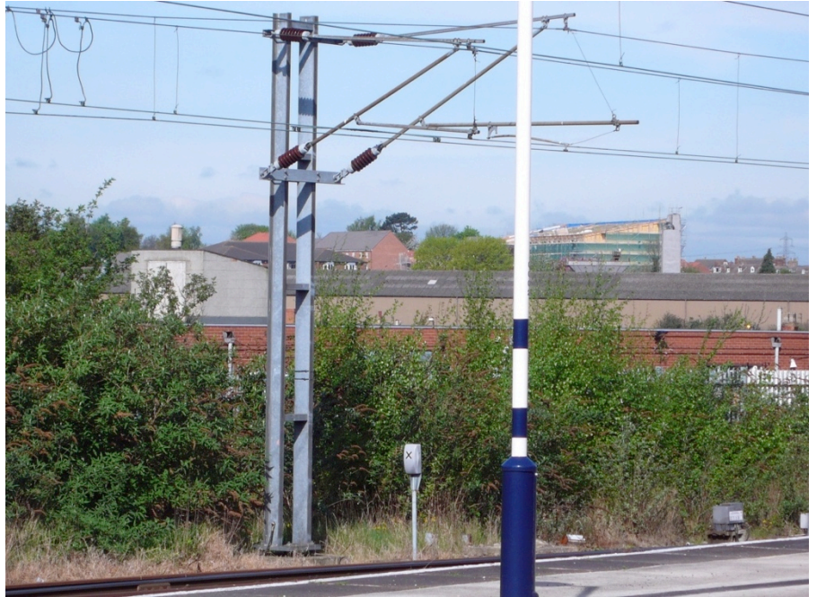
Figure 2-1 View of construction from Grantham Station. 29 April 2010.
