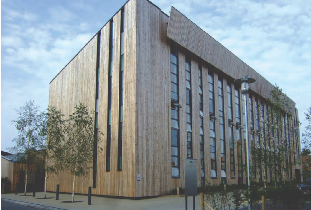
Figure 2-3 North facade of the Woodland Trust HQ. The roof slopes down to the south to accommodate future photovoltaic panels
