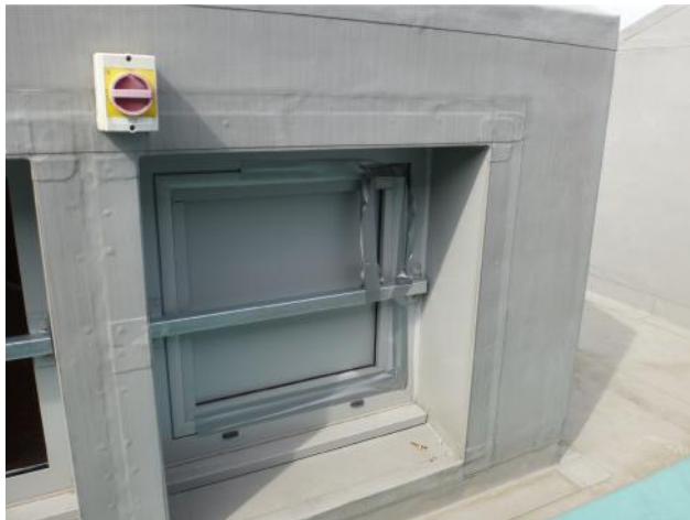
Incubator unit vent taped-up
