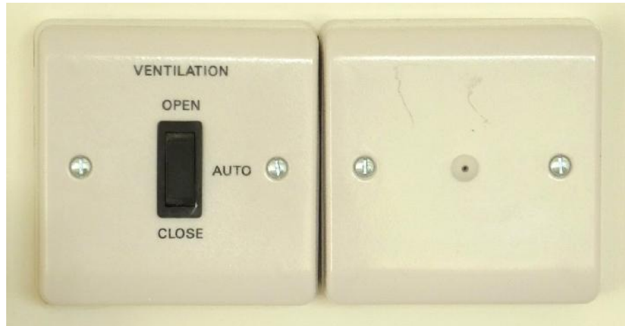
Ventilation controls (momentary open/close switch) and temperature sensor
