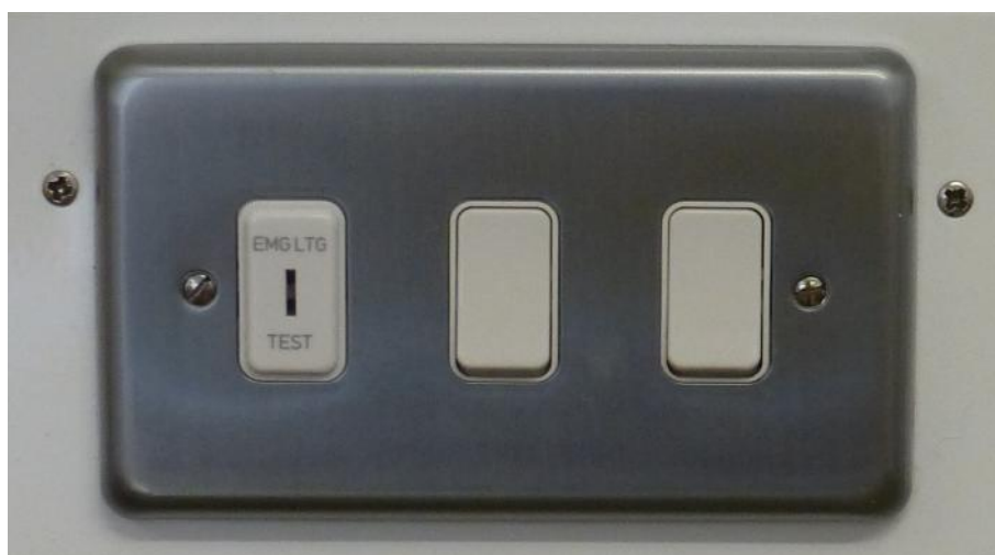
Momentary on/off light switches, push and hold to dim
