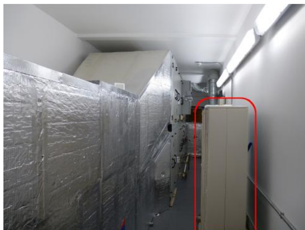
Condenser unit located in unventilated plant room
