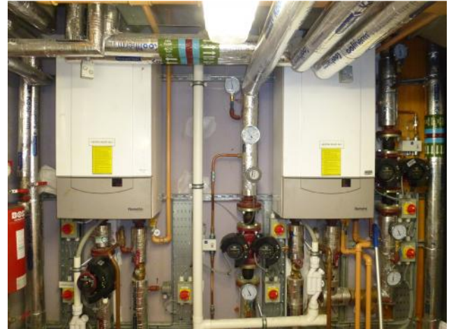
Identical boilers serving separate space heating and DHW circuits
