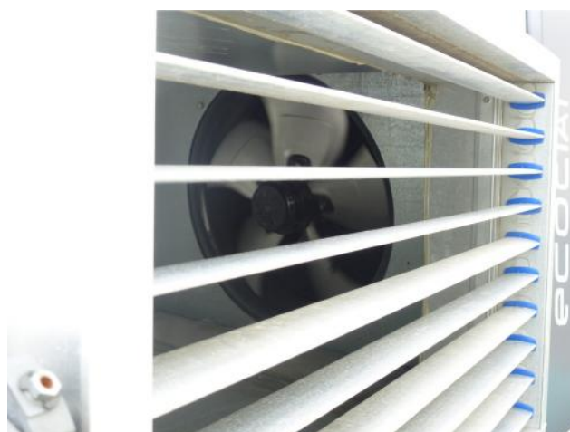
Motorised damper prior to replacement
