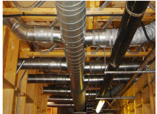
Main extract duct and connections to extract terminals
