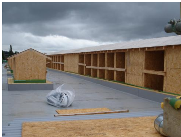
Roof level ventilation terminals during construction
