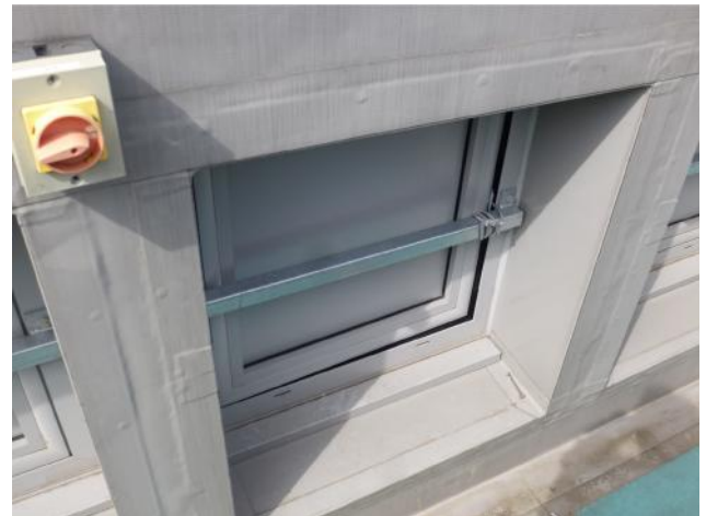
Incubator unit vent tied closed
