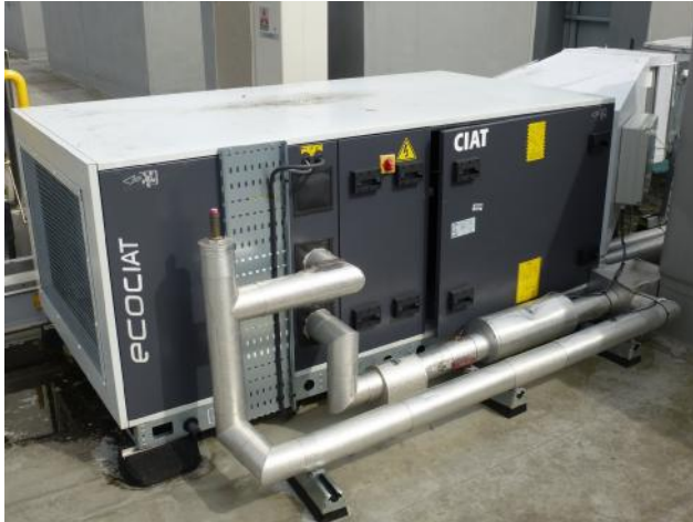
Roof-mounted exhaust-air heat pump (EAHP)
