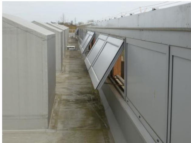
Only four of six vents on one side of the street were opening properly
