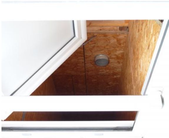
View into natural ventilation shaft showing mechanical extract terminal
