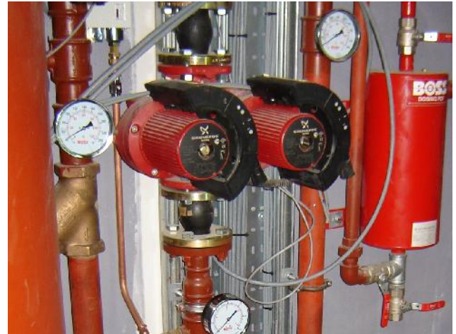
Secondary circuit pump, serving building heat emitters
