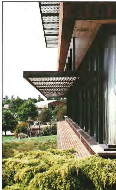
Typical office windows with overhangs and sunscreens.
