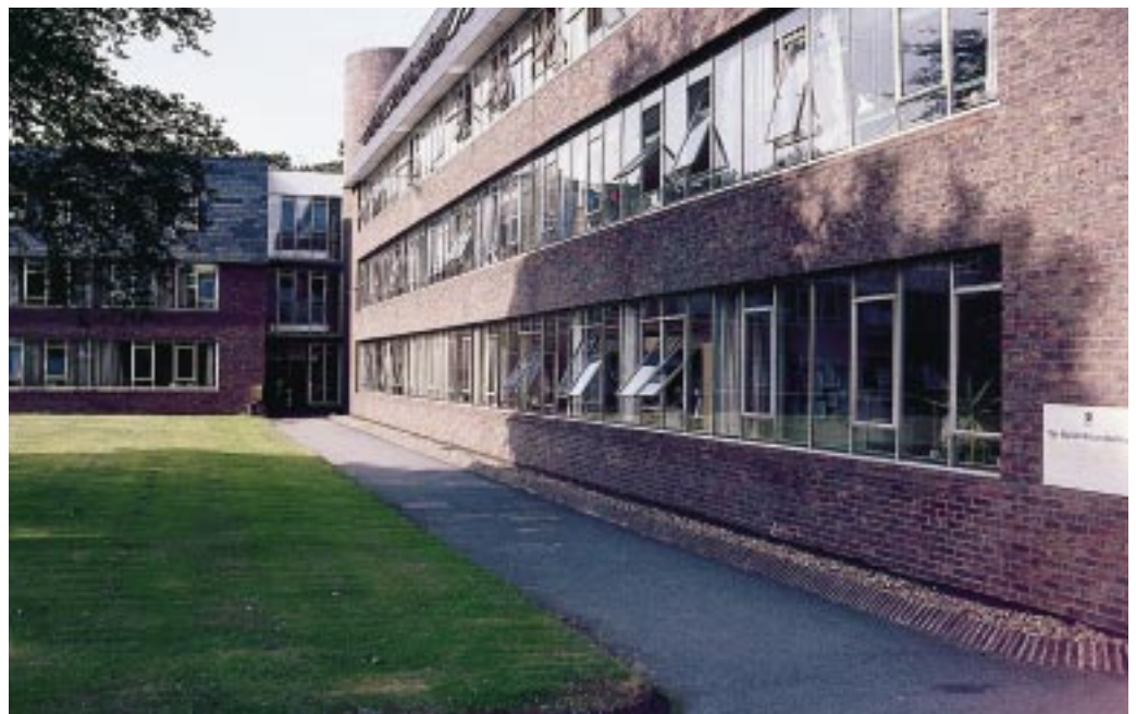
Figure 1 Typical elevation before refurbishment
