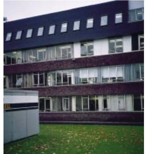
Figure 3 Modified windows in pilot scheme on the second floor
