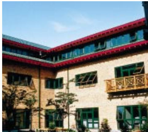
To meet property market requirements, this office, pre-let to The Body Shop, had to be capable of being AC. Its contingency design has plant, riser and ceiling void space for a variable air volume (VAV) system. However, with overhangs to shade the summer sun, careful window design, and energy-efficient lighting, its offices work well with natural ventilation alone.
